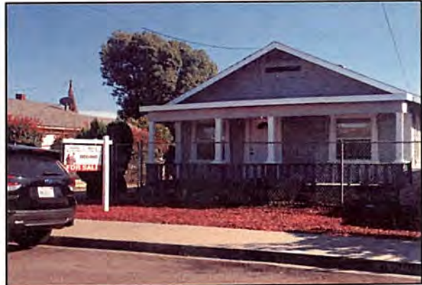
OCT/2021 - INSPECTION PHOTO
