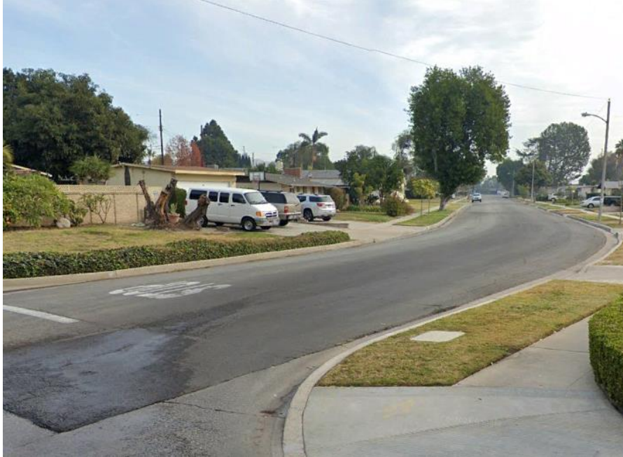
Gregory Ln – Pre-Construction Condition (from Google Earth, December 2020), facing North East
