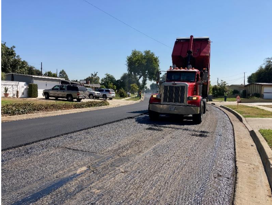
Gregory Ln – Placing Asphalt, facing East
