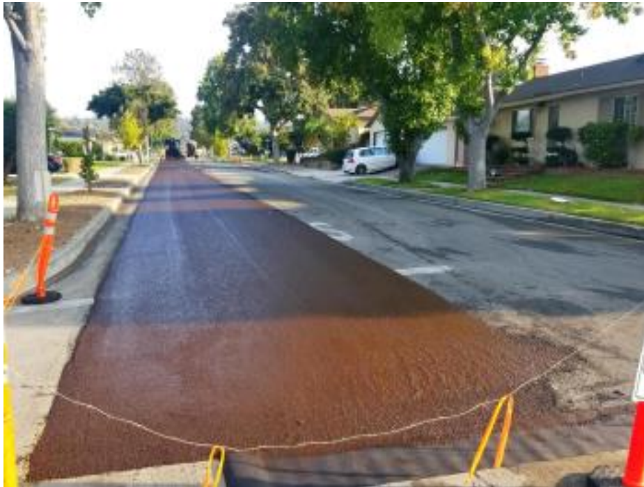
Kinley St – Slurry Seal Application, facing North
