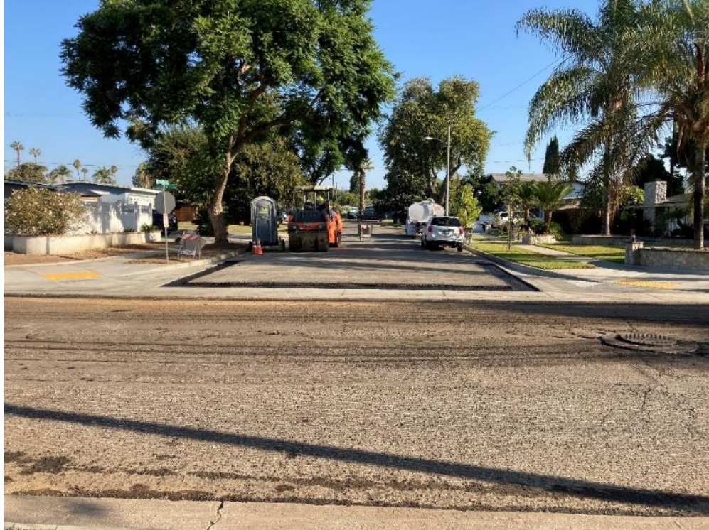
Gregory Ln and Chantry Dr – Paving Preparation, facing North
