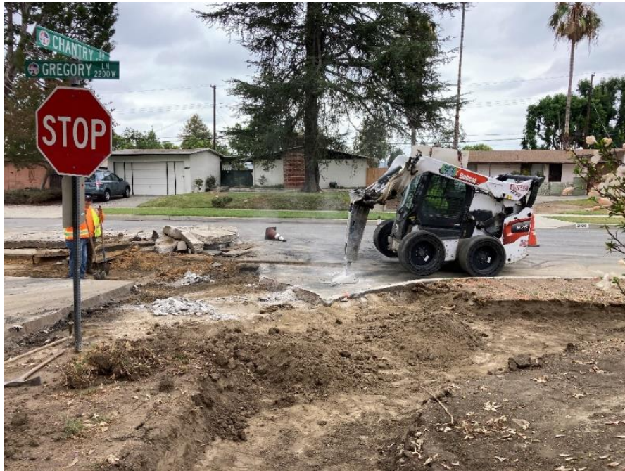
Gregory Ln and Chantry Dr – Concrete Demolition, facing South
