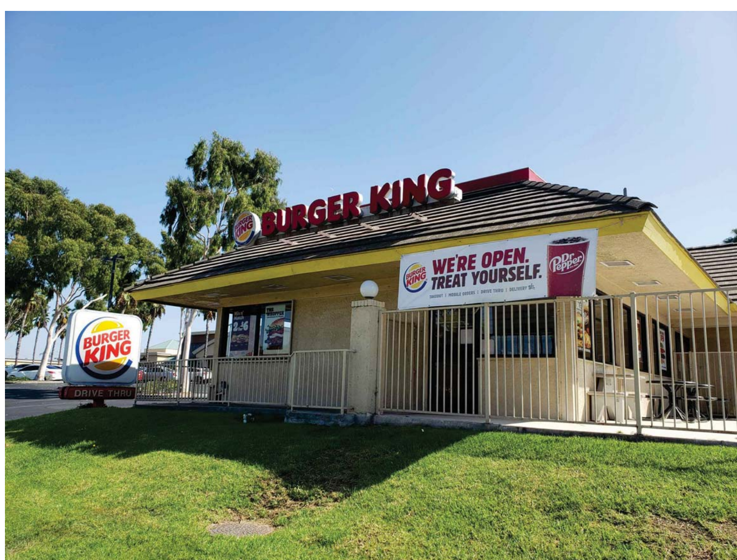
NORTH ELEVATION EXISTING CONDITIONS PHOTO
