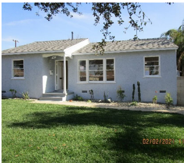
Code enforcement efforts leading to housing repairs.
