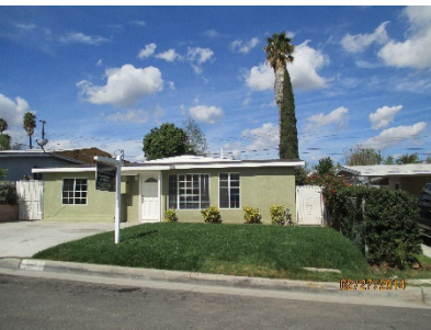
Before and after photos of code enforcement success
