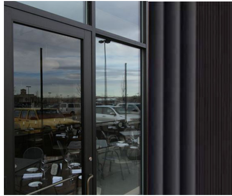
2 STOREFRONT BY: ARCADIA (2X6 AFG-601 SERIES) OR EQUAL MODEL: 2X6 AFG-601 SERIES OFFSET FINISH: BLACK ANODIZED, CLASS 1(AB-8)
