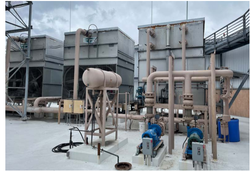
City of Anaheim, West Tower HVAC Replacement
