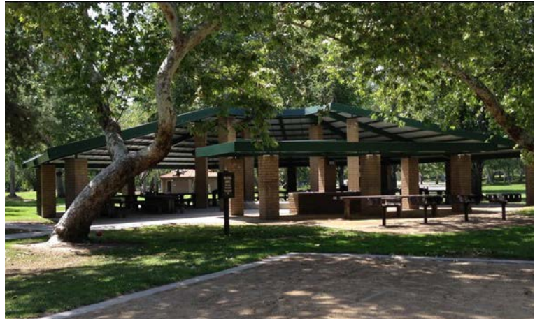
Irvine Regional Park Shade Structure
