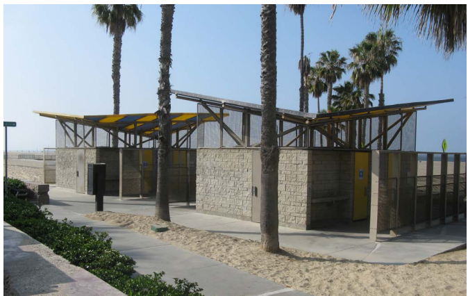
City of Santa Monica, Beach Restrooms 16 & 17
