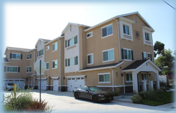
Coyote Creek Homes 506-510 S. Walnut Street
