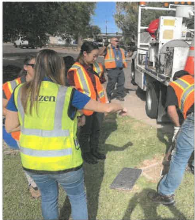
Hazen team members were on-site with Utility staff to test out a utility-owned industrial vacuum truck prior to hiring a third party contractor.
