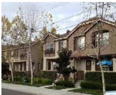
Multi-Family Housing, Brea
