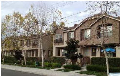
Multi-Family Housing, Brea
