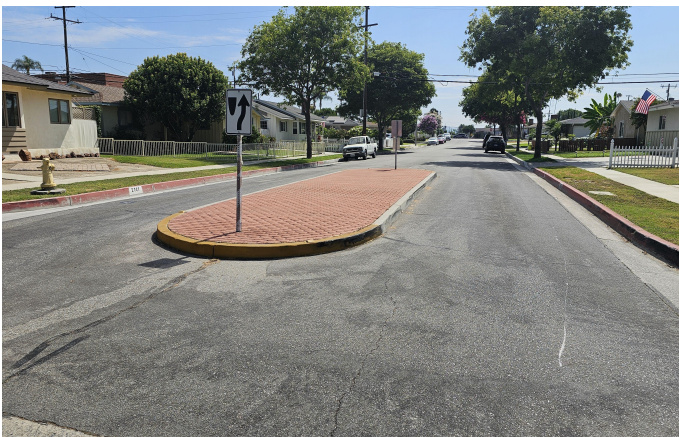
Raised Median Island
