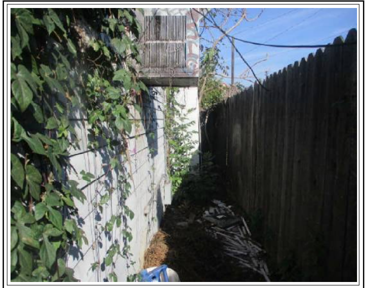
Rear of Unit 2
