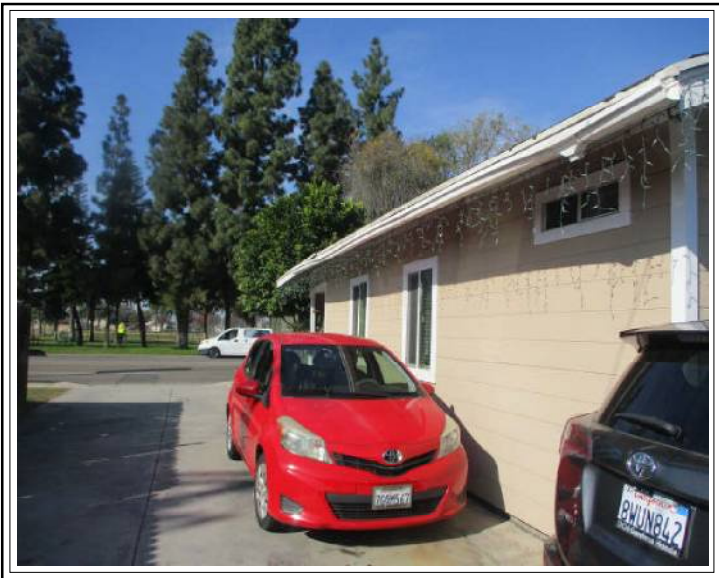
Side of Unit 1/Driveway
