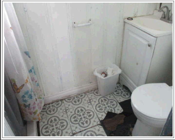
Bathroom in Unit 2
