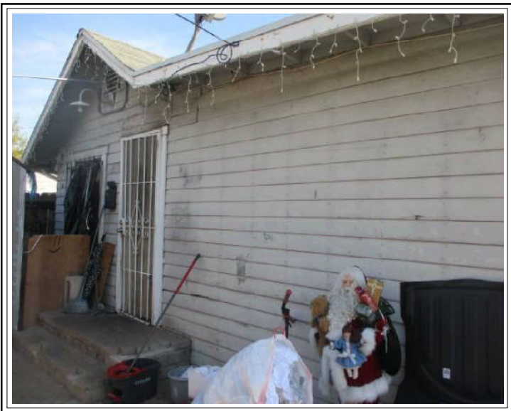
Front of Unit 2
