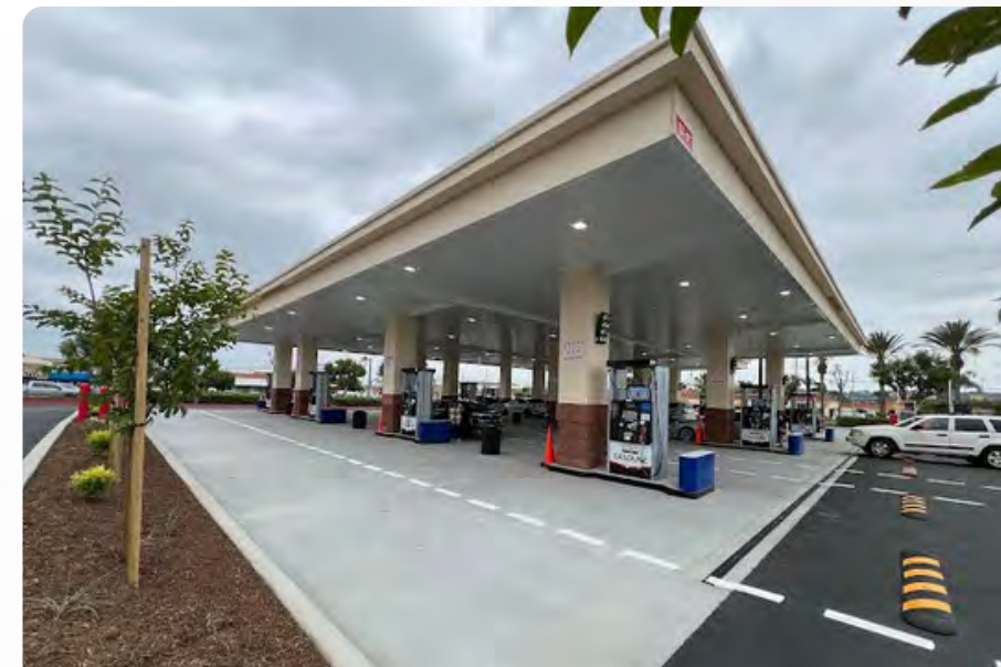
Costco Gasoline Expansion 103 N. Beach Blvd.
