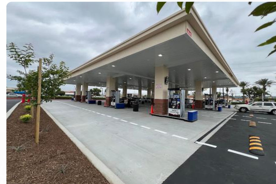
Costco Gasline Expansion 103 N. Beach Blvd.
