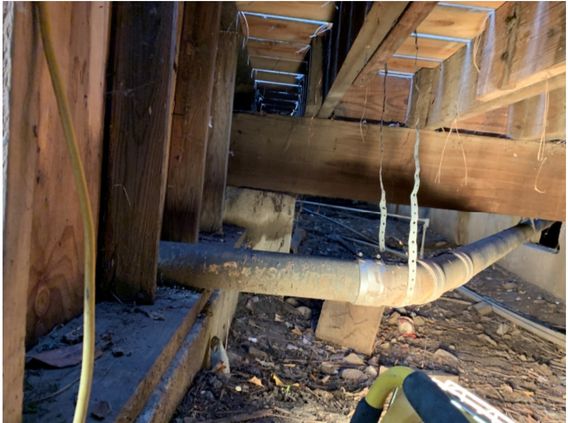
Photo 24– Exterior Decks – Framing.
