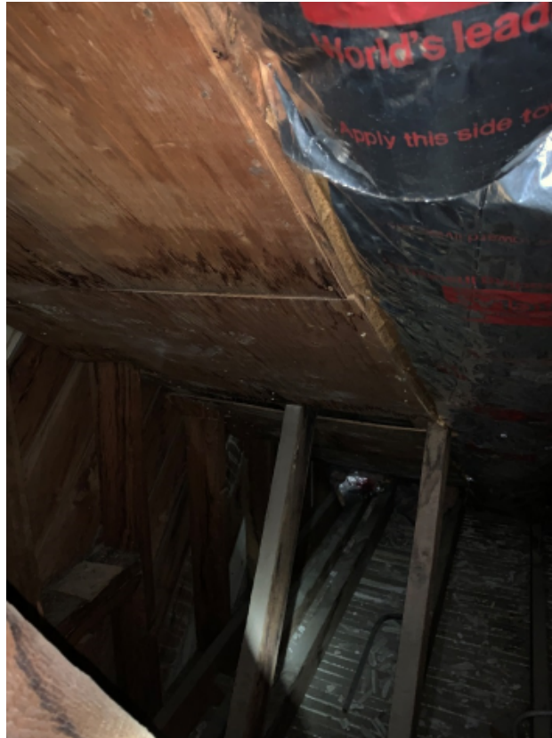
Photo 2 – Area A – Attic Crawl Space.
