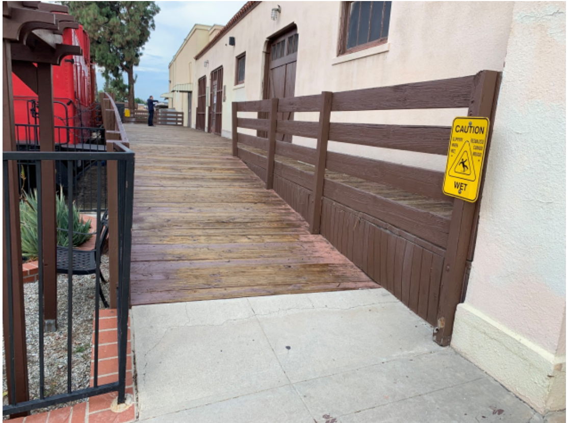
Photo 27– Exterior Decks – Ramp
