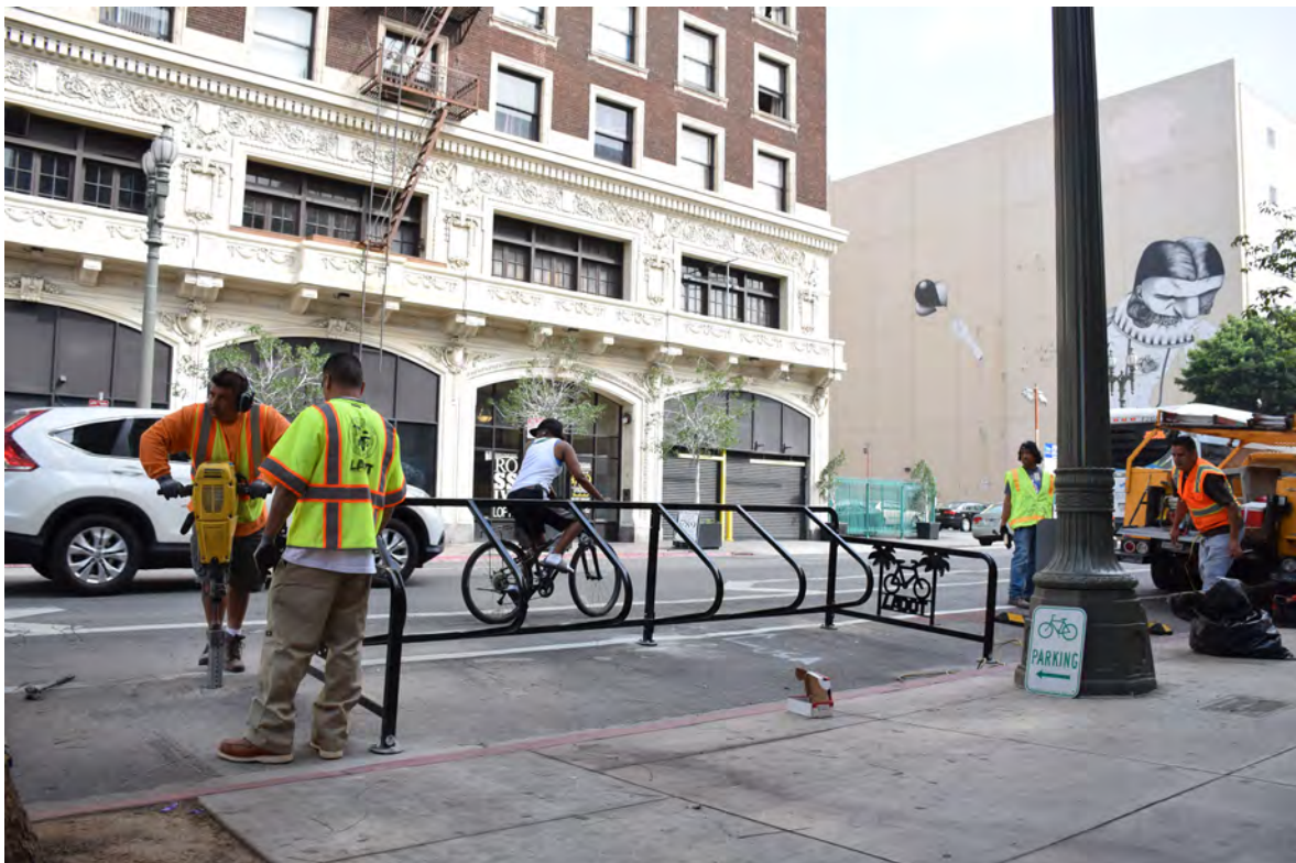
Bike Corral Installation at 5th St and Main St
