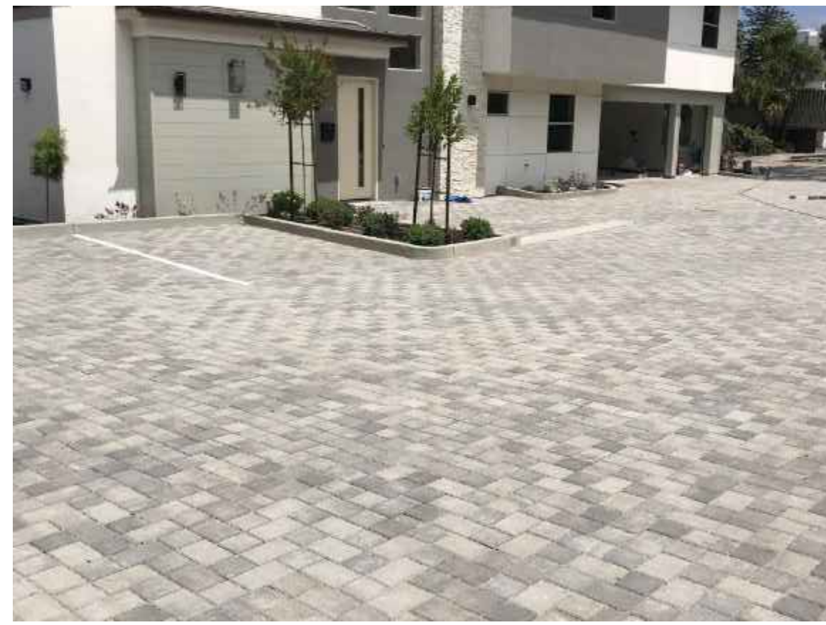
11. PROPOSED PERMEABLE PAVERS WITH 3-PIECE MODULAR SYSTEM BY BELGARD COMMERCIAL OR APPROVED EQUAL. "COLOR TO BE LIGHT GRAY MATCHING DESIGN ELEVATION'S GRAY COLOR"
