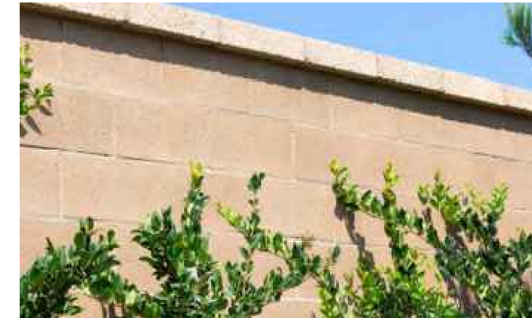
9. PROPOSED 6" WIDE PRECISION CMU BLOCK WALL SURROUNDING THE PROPERTY FOR 3'-0" & 6'-0" HIGH WALL WITH 2" CAP BY ORCO BLOCK OR ANGELUS BLOCK OR APPROVED EQUAL WITH "TAN-BROWN COLOR"
