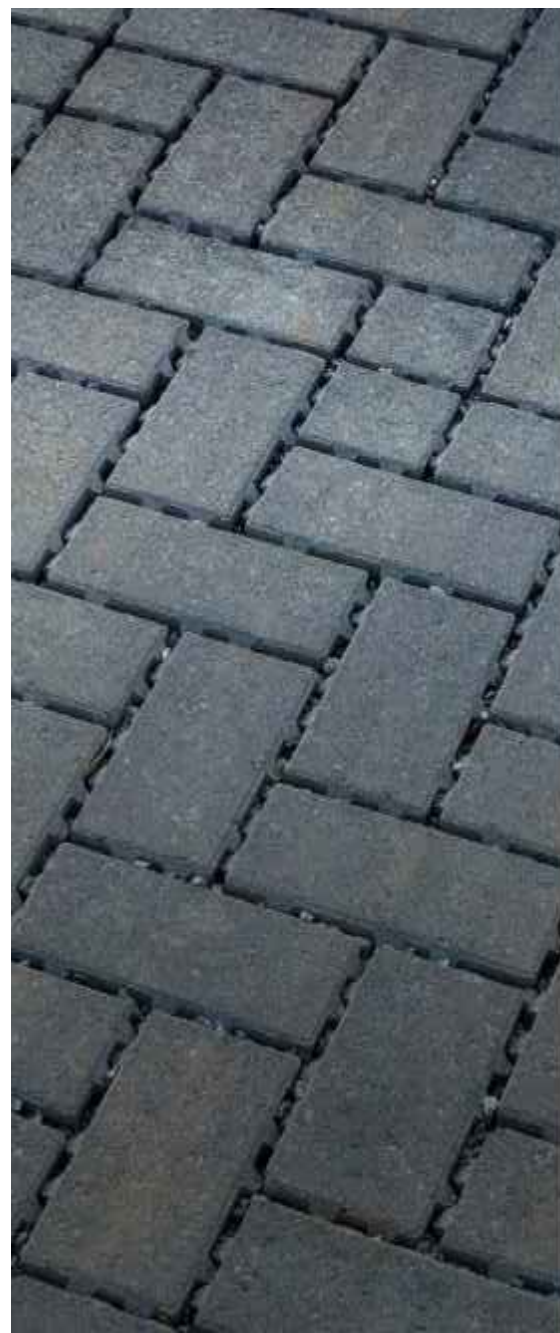
11. PROPOSED PERMEABLE PAVERS WITH 3-PIECE MODULAR SYSTEM BY BELGARD COMMERCIAL OR APPROVED EQUAL. "COLOR TO BE LIGHT GRAY MATCHING DESIGN ELEVATION'S GRAY COLOR"
