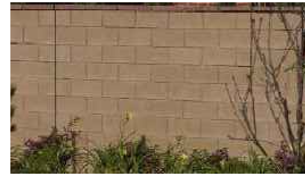
9. PROPOSED 6" WIDE PRECISION CMU BLOCK WALL SURROUNDING THE PROPERTY FOR 3'-0" & 6'-0" HIGH WALL WITH 2" CAP BY ORCO BLOCK OR ANGELUS BLOCK OR APPROVED EQUAL WITH "TAN-BROWN COLOR"
