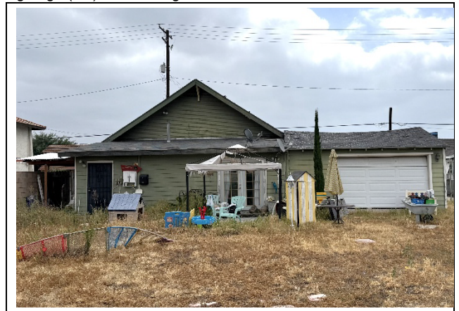
Image 4: Attached garage and rear addition, west elevation, view facing east. Source: GPA, June 2025.
