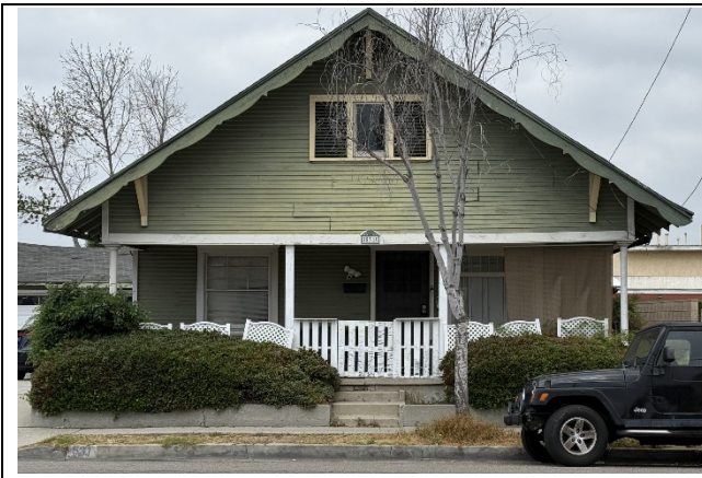
Image 1: East (primary) elevation, view facing west. Source: GPA, June 2025.
