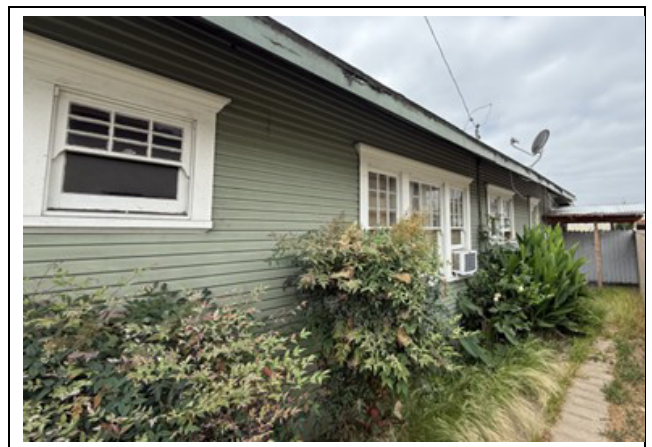
Image 6: North elevation, view facing southwest. Source: GPA, June 2025.
