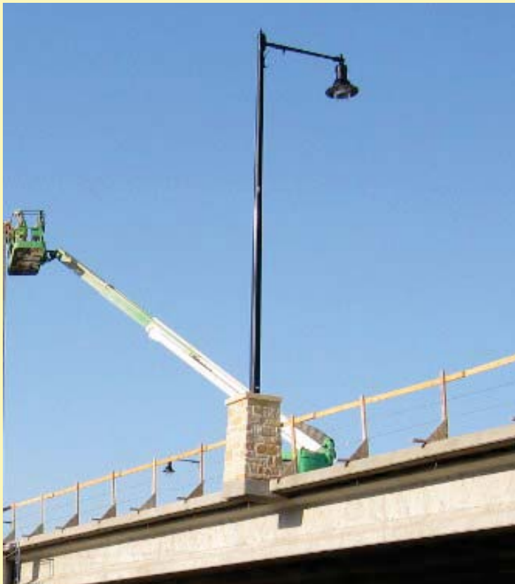
Electricians are installing the bridge lighting.
