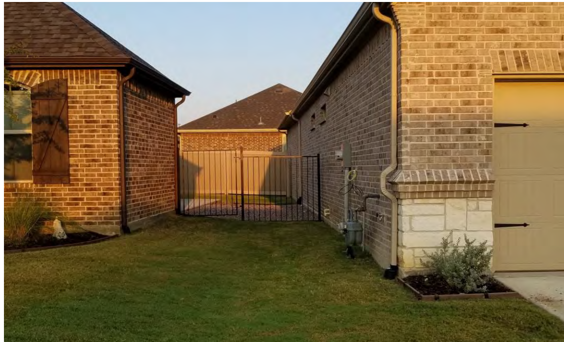
The picture to the right shows the front fencing detail, which all have an access gate at the front and rear. This also shows how the rear privacy fence is part of these particular homes, which “back up” to other homes.
