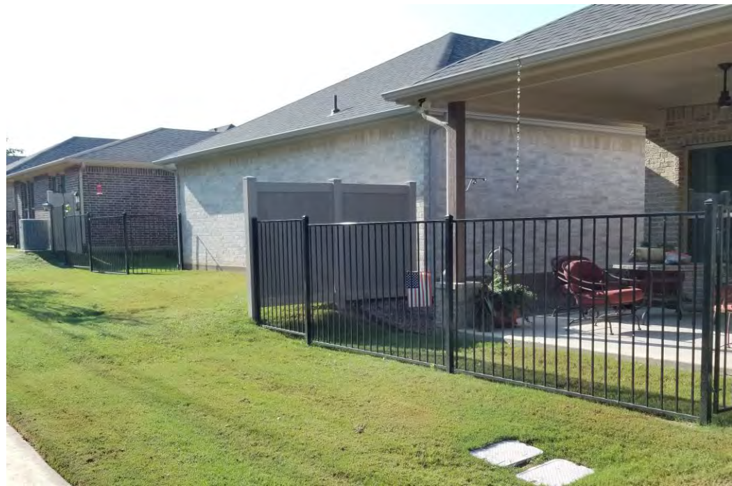
The picture to the left shows where Privacy fence is used between homes that back up to viewpoints, also showing how the Wrought Iron fence is used for visibility to the same areas.
