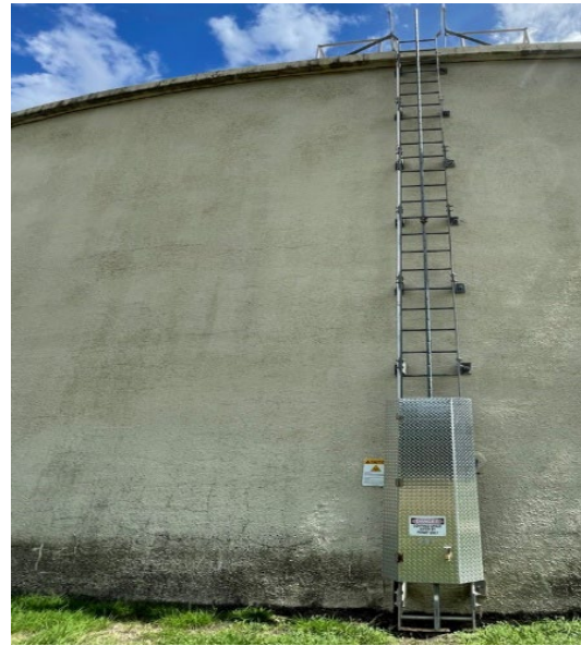
Photo No. 36 Exterior Ladder – Fall Protection
