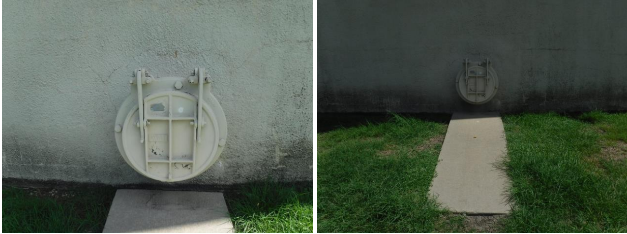
Overflow flapper and splashpad
