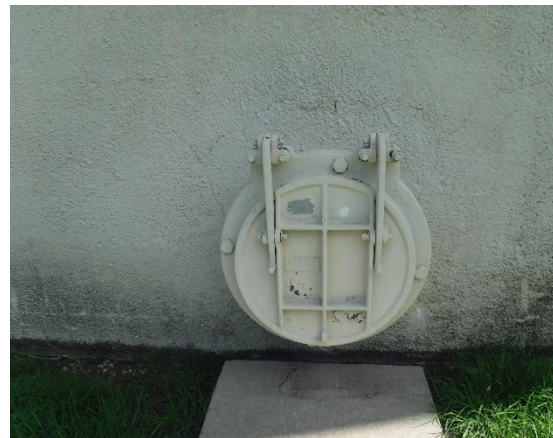
Photo No. 52 Overflow flapper
