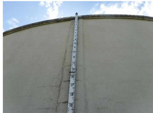
Photo No. 17 Liquid Level Indicator for water depth
