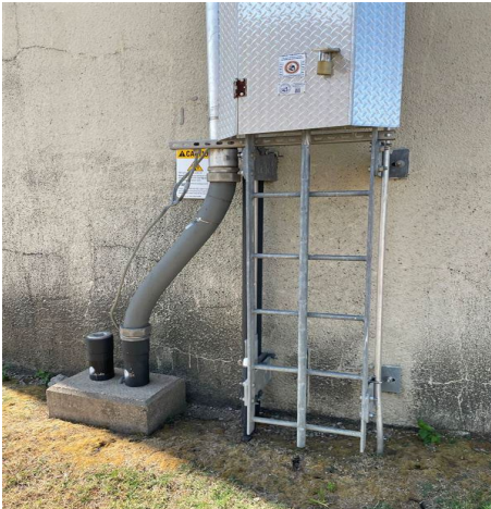
Photo No. 37 Exterior Ladder– Fall Protection and Ladder Guard
