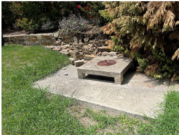
Photo No. 58 Storm Drain inlet on West W/ damaged landscape
