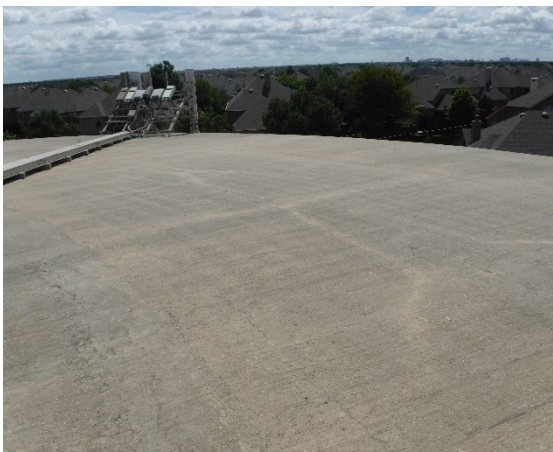
Photo No. 10 Cracks at Roof Slab (Exterior)
