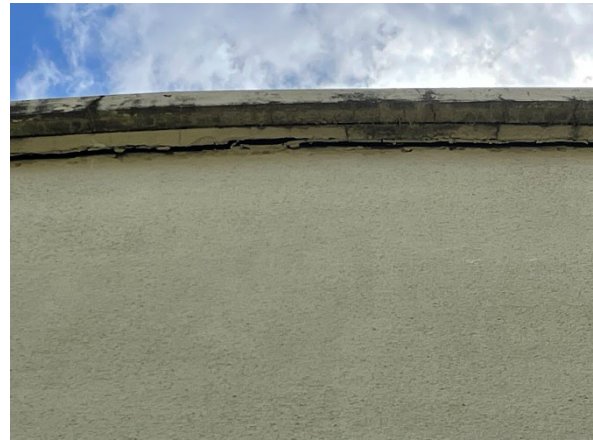
Photo No. 19 Gap between roof slab and wall
