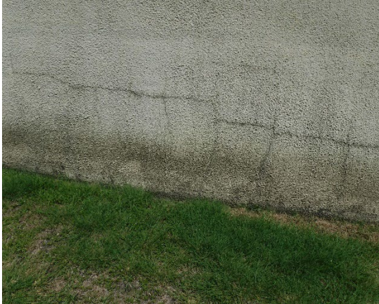
Photo No. 18 Possible Cracks Forming
