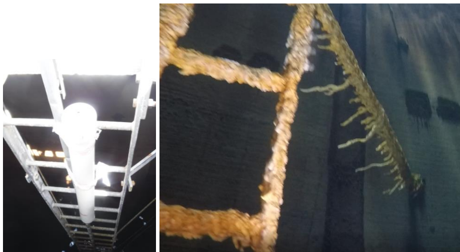
Inside Ladder growth on lower ladder
