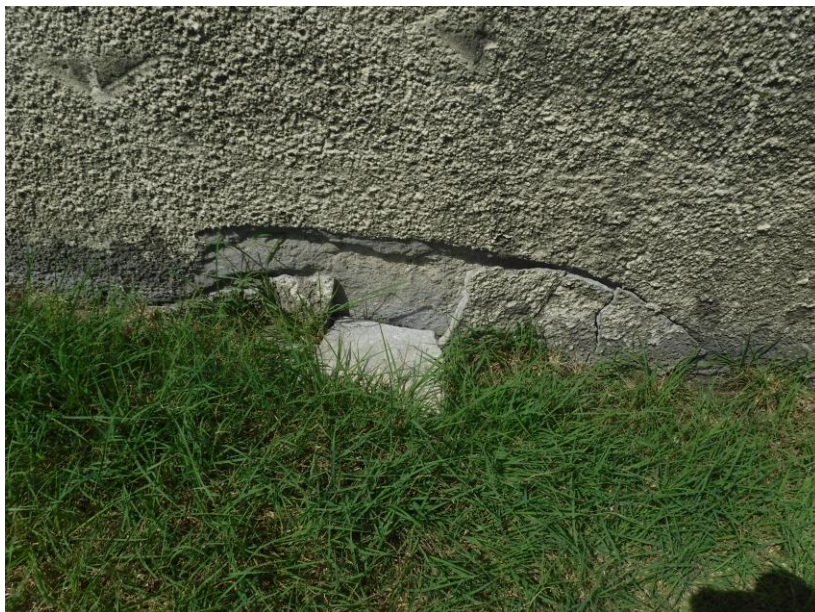
Side of tank with some chipped texture
