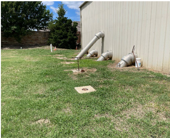
Photo No. 70 Outlet pipe from tank to Pump House
