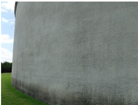
Photo No. 20 Discoloration observed at bottom of the walls
