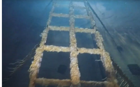
Photo No. 40 Interior Ladder Corrosion
