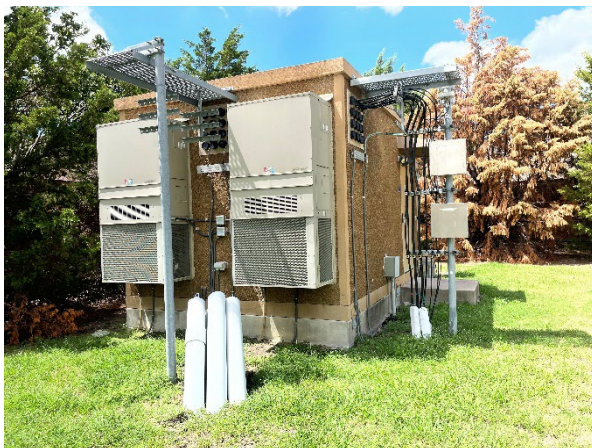
Photo No. 60 Incoming wires to ATT building
