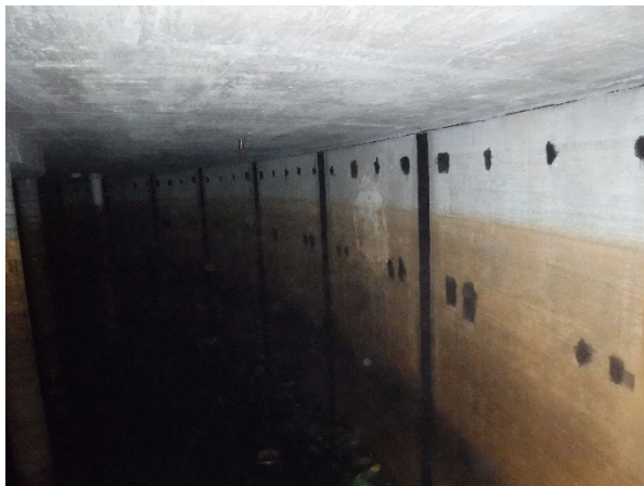
Photo No. 4 High rust deposit on interior surface of tank
