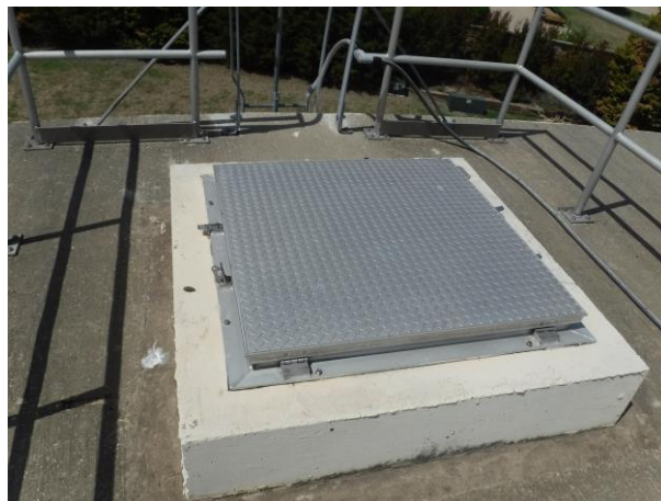
Roof Hatch closed
