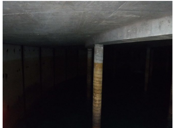
Photo No. 5 High rust deposit on interior column of the tank
