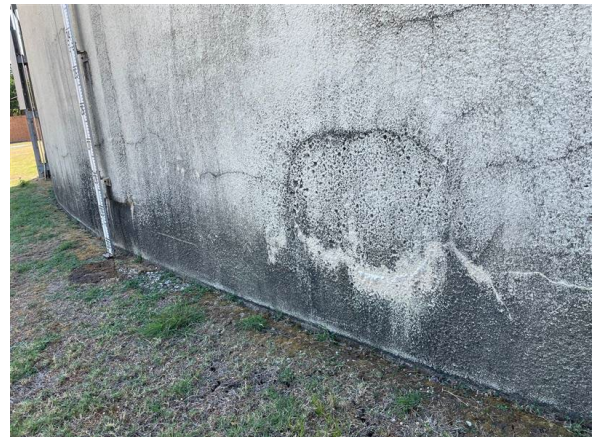
Photo No. 28 Manway from outer wall - Closed
