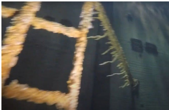
Photo No. 41 Biological Growth below water line
