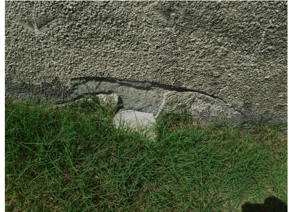
Photo No. 26 Spalling of Concrete
