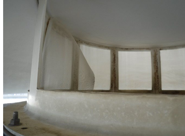
Photo No. 54 Damaged Roof Vent Screen
