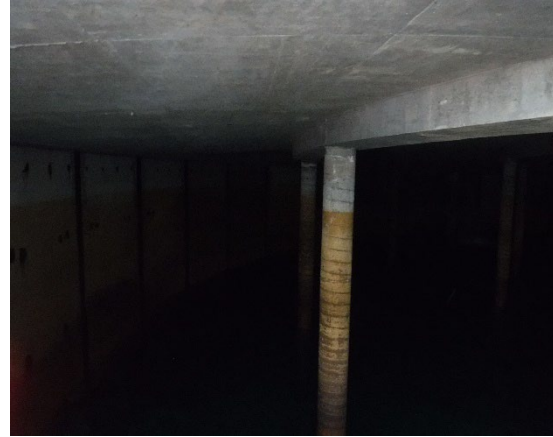
Photo No. 15 Interior Roof beam in good condition
