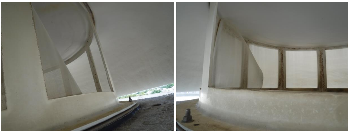
Top vent screen needs to be replaced
