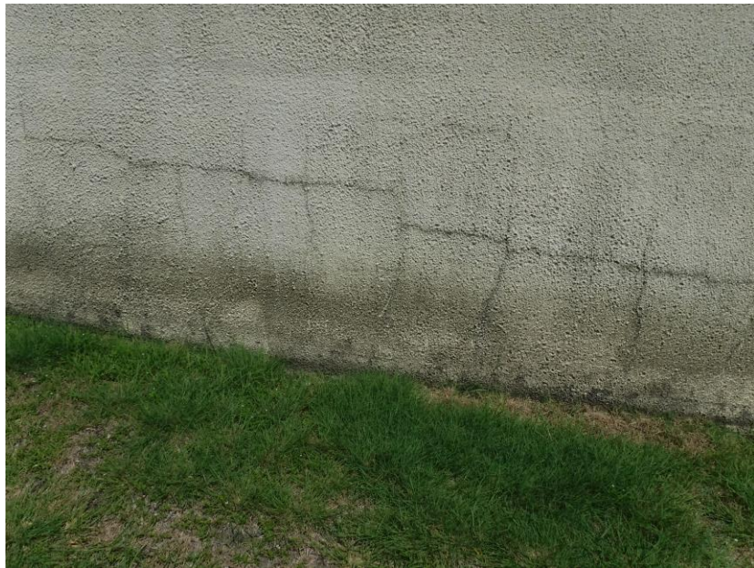
Side of tank with cracking in the texture
