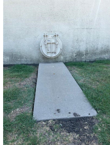
Photo No. 50 Overflow flapper and splashpad
