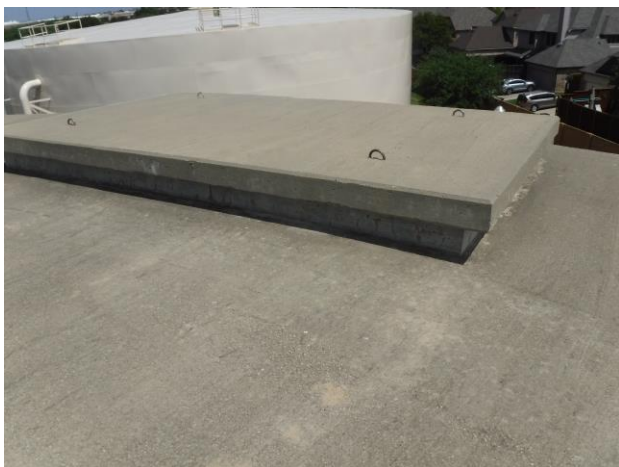
Roof of tank and concrete hatch
