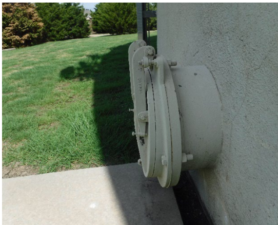
Photo No. 51 Overflow flapper side view
