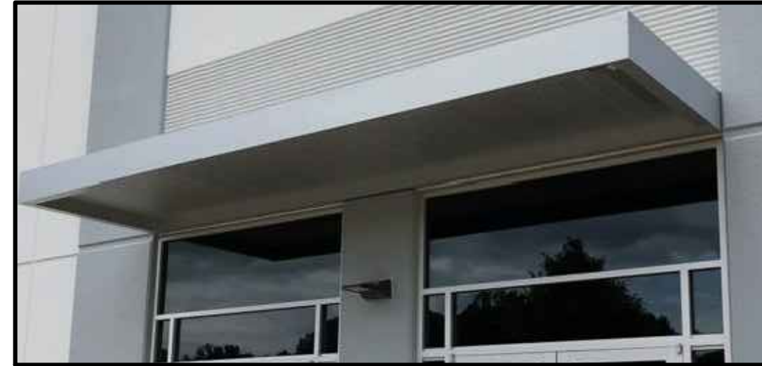
CANTILEVERED METAL AWNING: COLOR: NATURAL ALUMINUM
