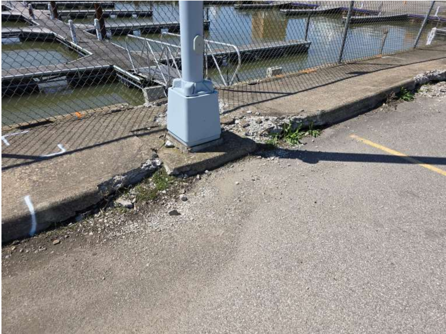
Lorain Engineering - Lorain Harbor Boat Club - replace 7
