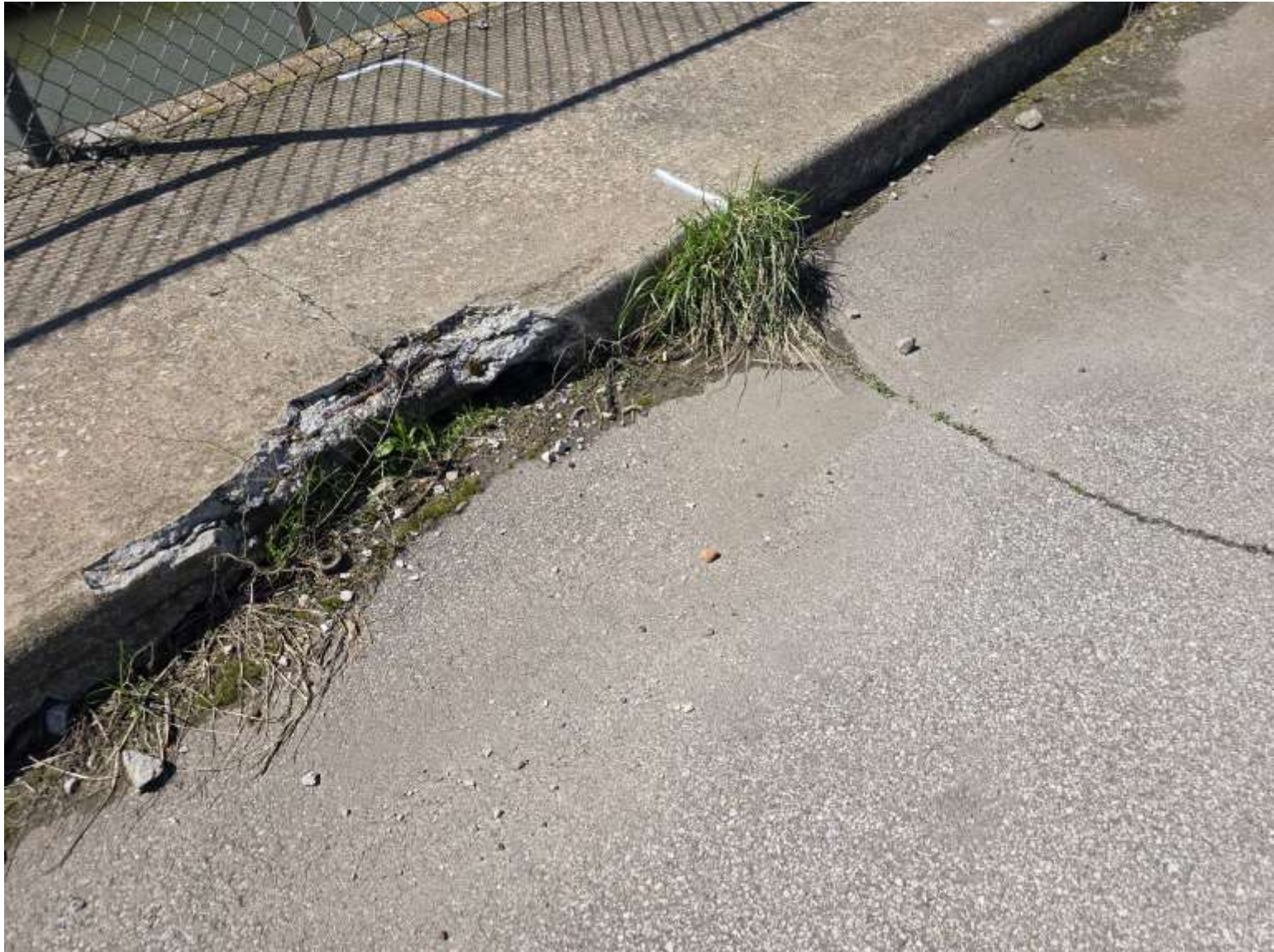
Lorain Engineering - Lorain Harbor Boat Club - replace 6
