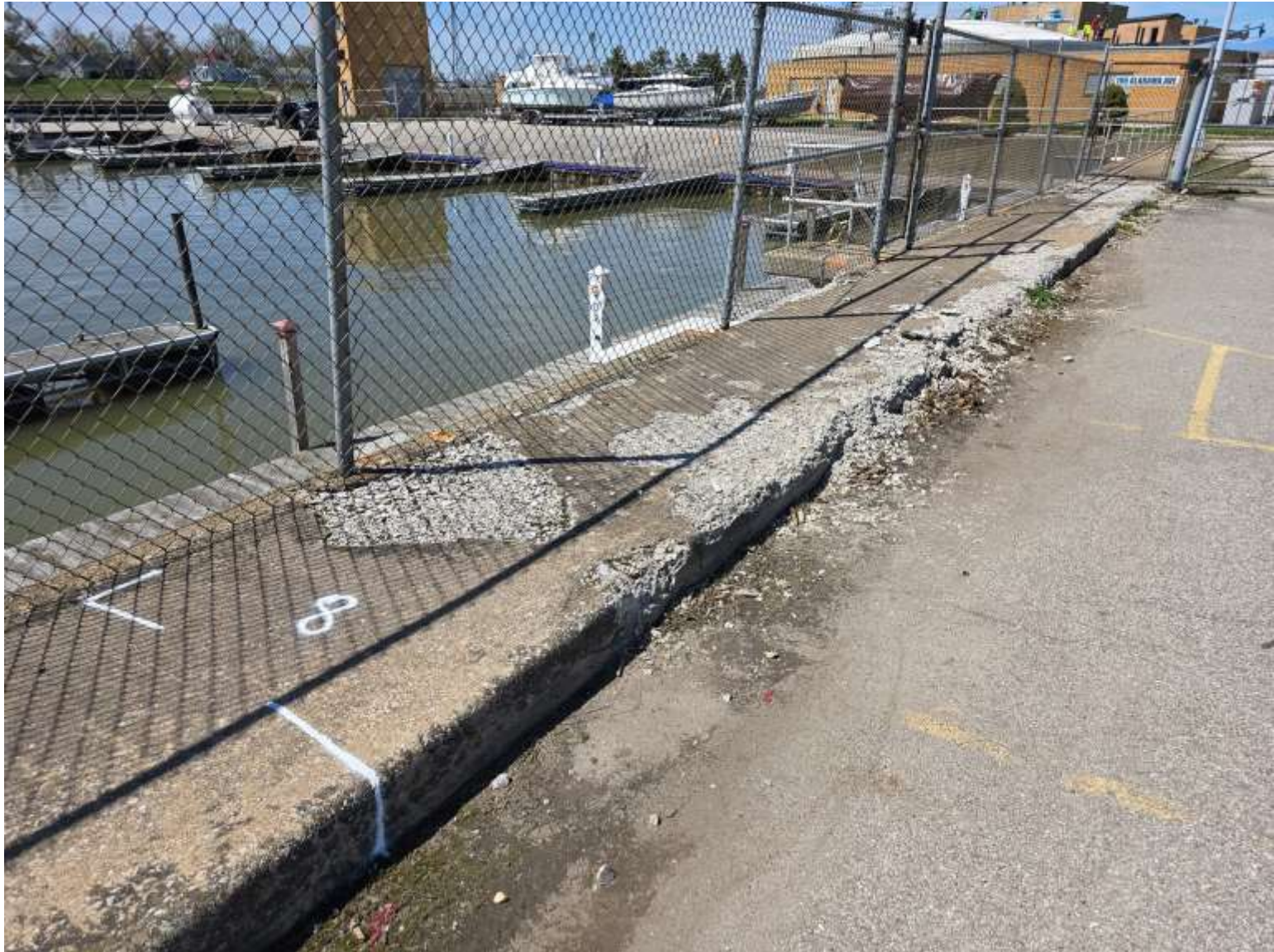
Lorain Engineering - Lorain Harbor Boat Club - replace 8
