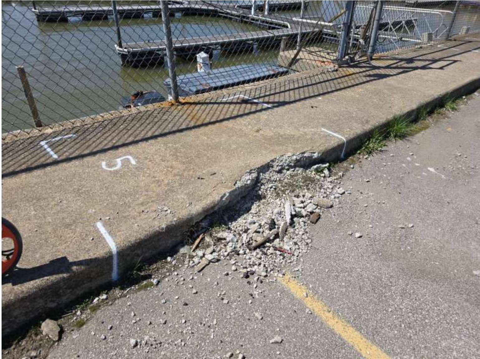
Lorain Engineering - Lorain Harbor Boat Club - replace 5
