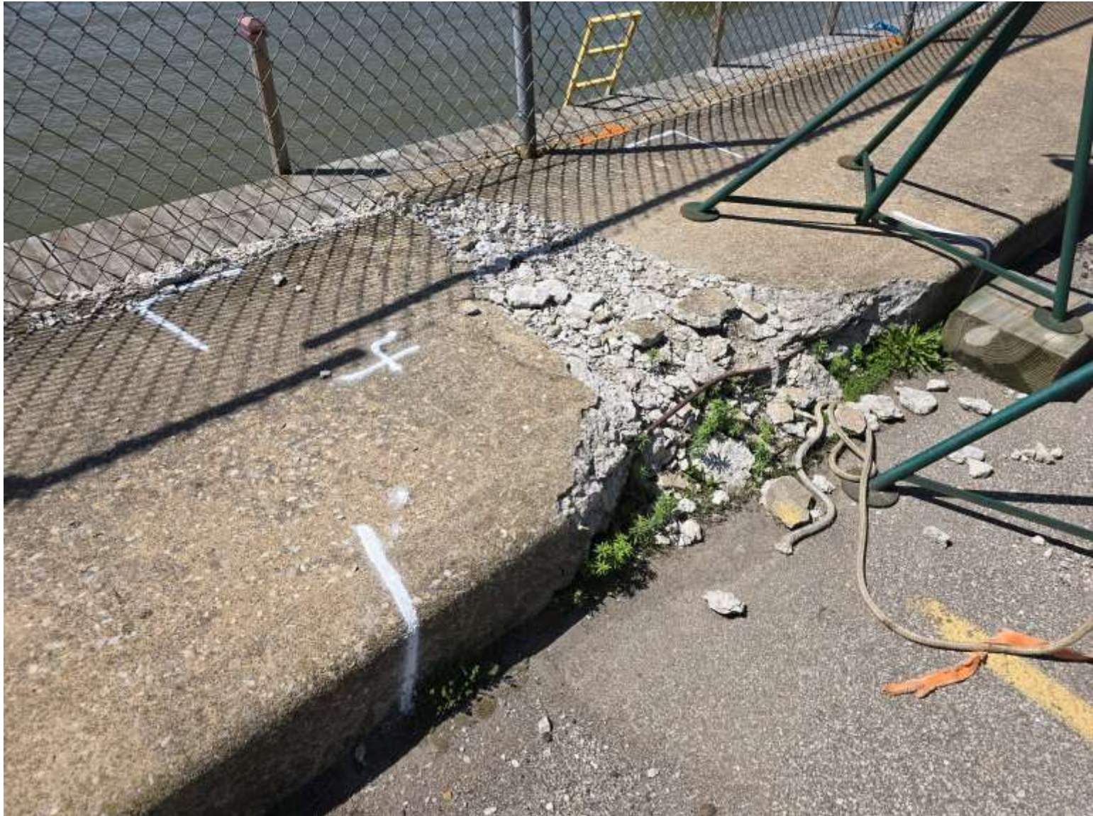
Lorain Engineering - Lorain Harbor Boat Club - replace 4
