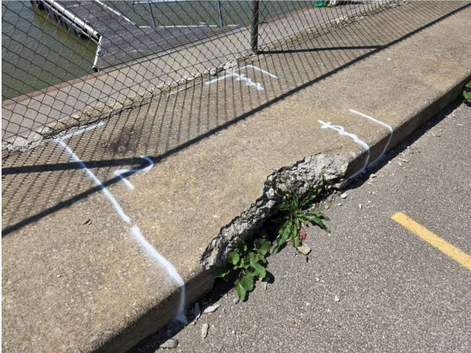
Lorain Engineering - Lorain Harbor Boat Club - replace 2
