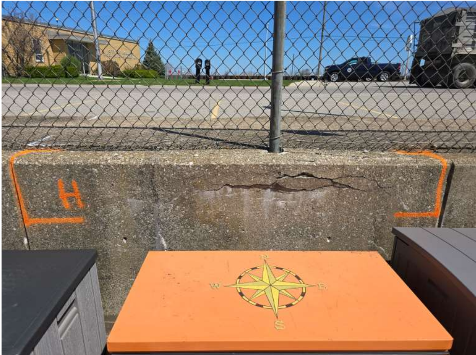
Lorain Engineering - Lorain Harbor Boat Club - patch H
