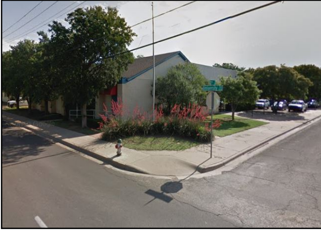
University Avenue and 25 th Street looking northeast.
