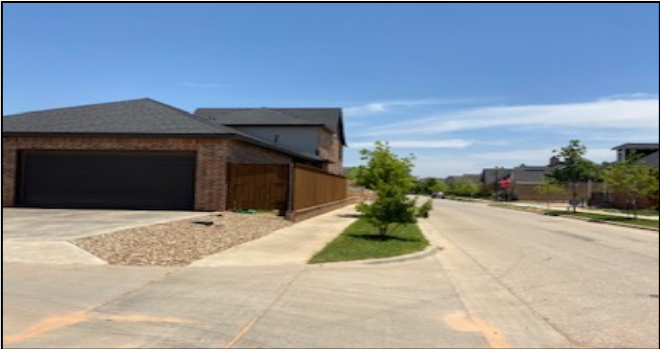
North view on west side
