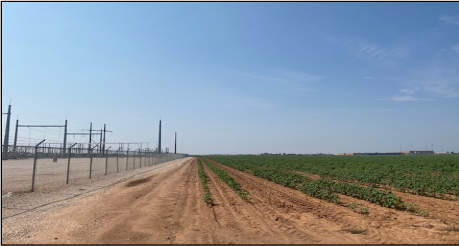
Subject property. View to the south.
