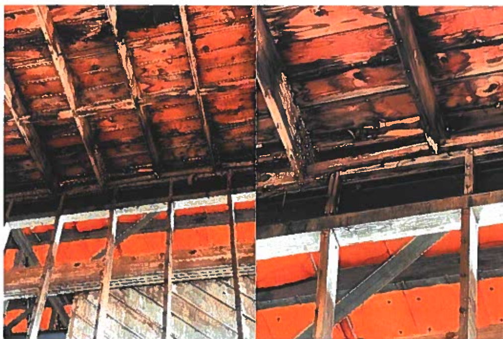
Figure-2-10: Compromised Roof Structure
