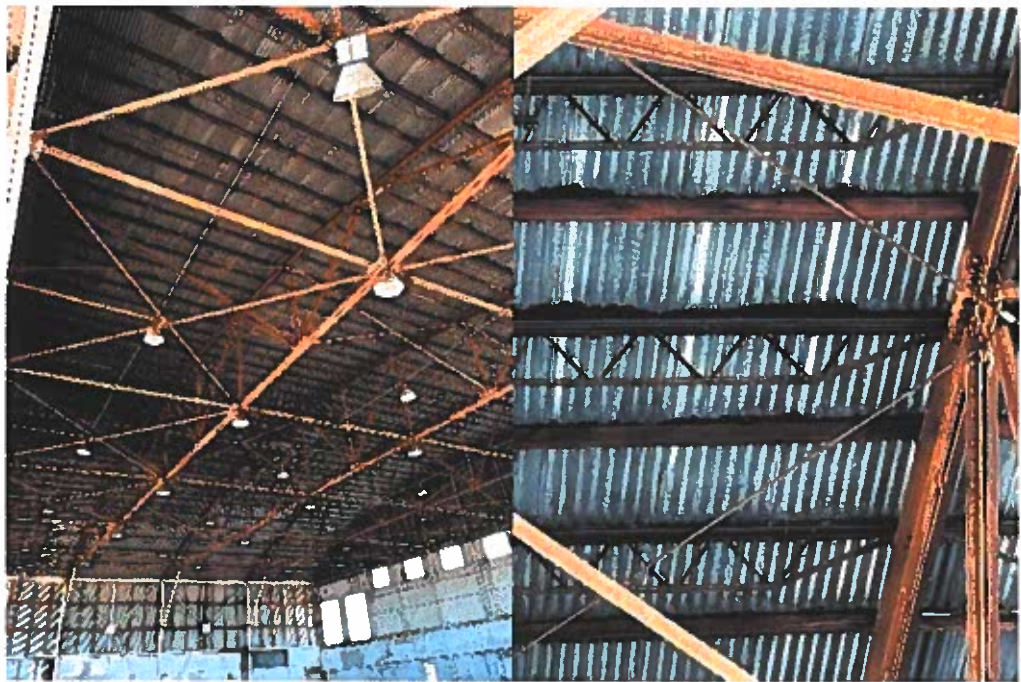
Figure-2-2: Hangar West Roof Framing
