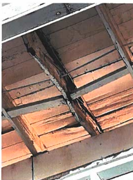
Figure-2-11: Compromised Roof Structure
