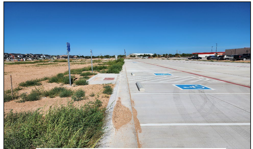
View to the north.
