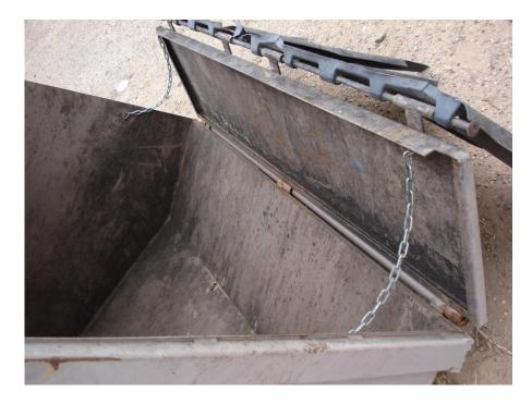
Chain attachment metal lids portion to side of dumpster.
