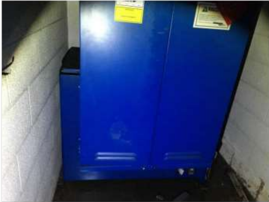
21 - Elevator hydraulic oil reservoir in 1212 Main Street
