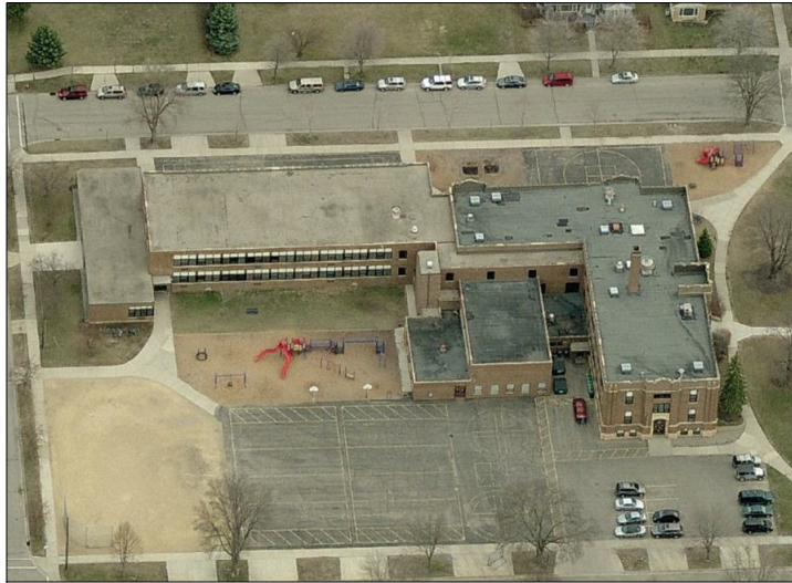
Roosevelt Elementary School 300 West Sixth St. Mankato, MN 56001
