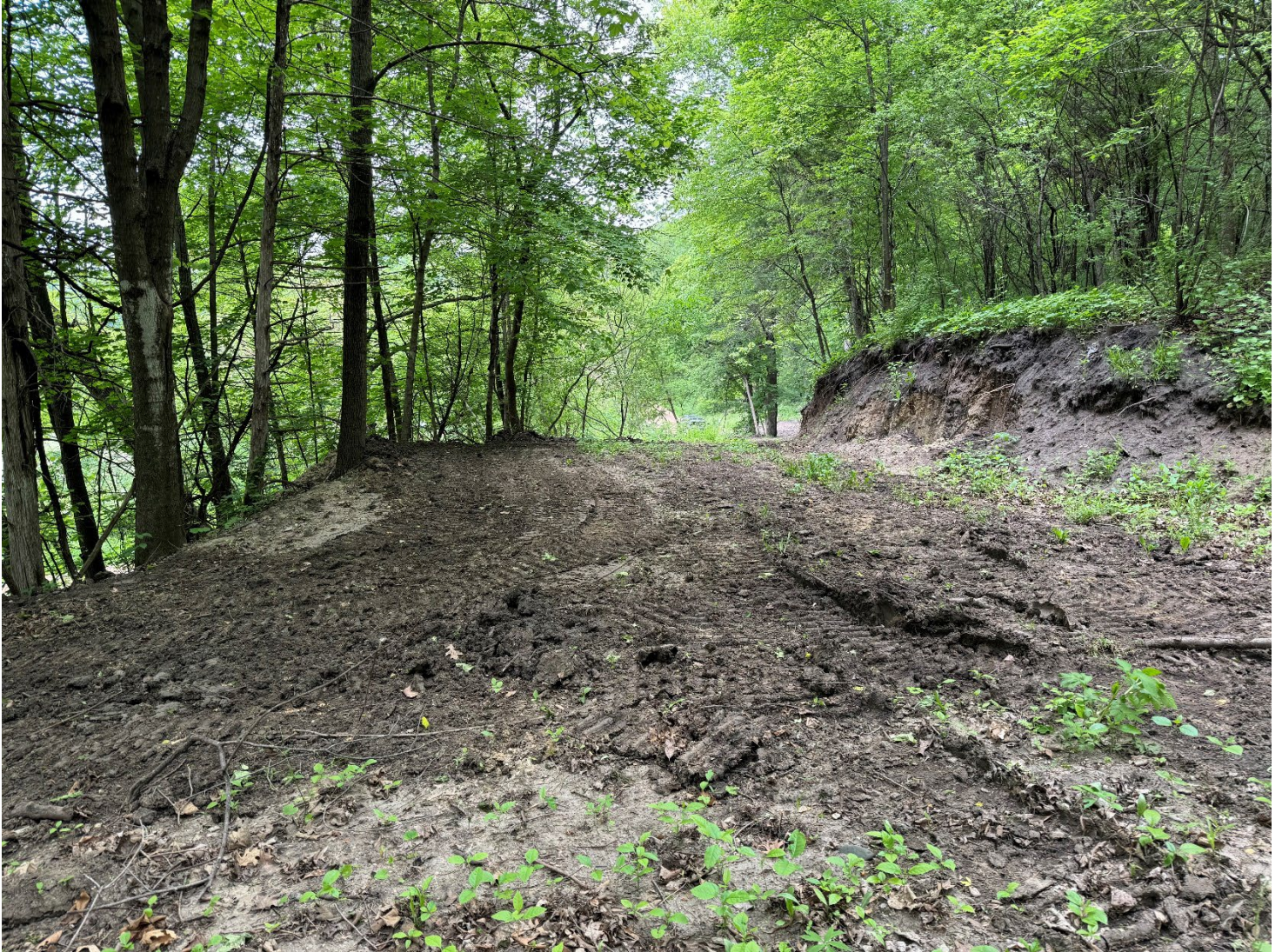
Machinery Tracks/Wide Shot- Picture 1
