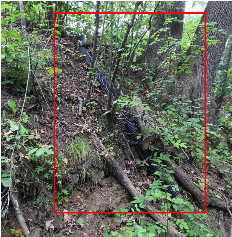
Figure 9. Drain Extending from House Partially Down the Slope Near Pool Area
