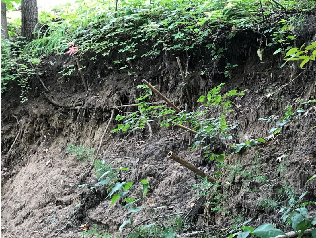
Figure 11. Potential Past Slope Stabilization Measure on Eastern End along the Peninsula
