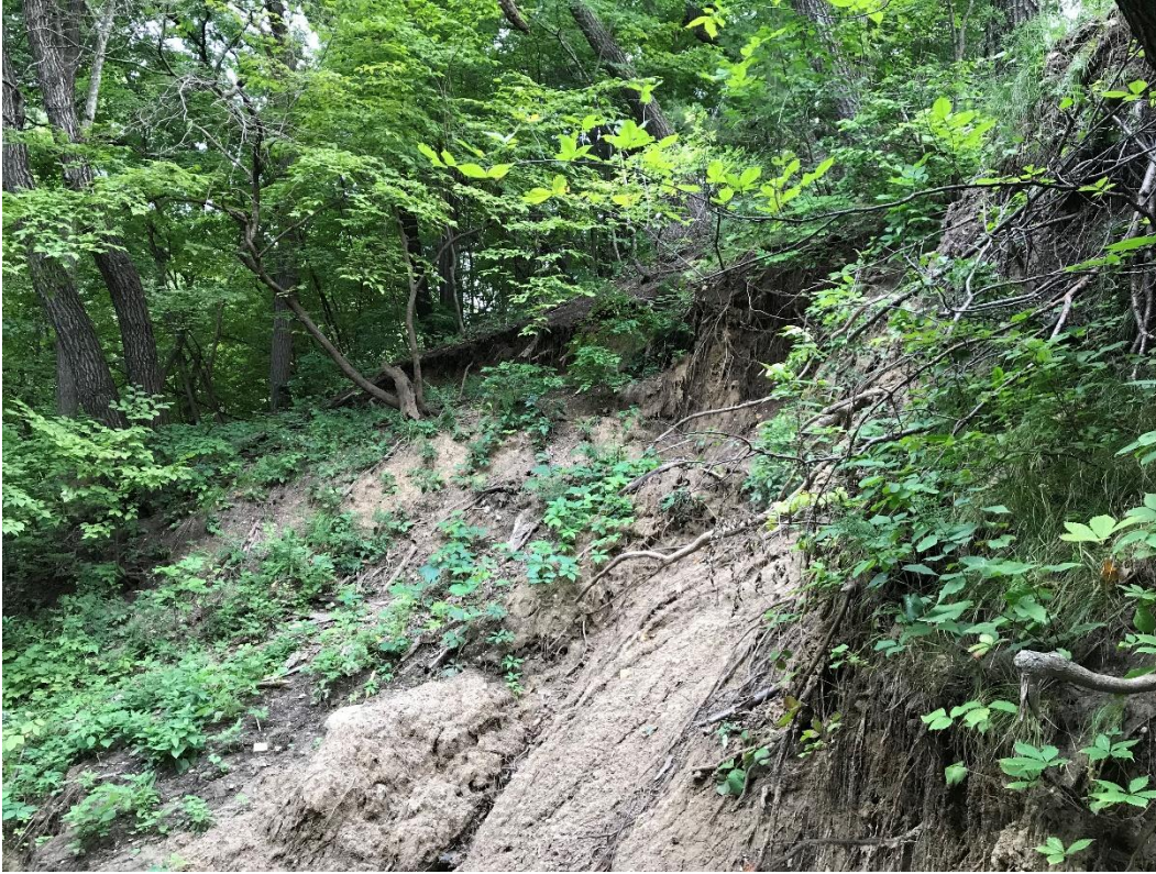
Figure 5. Observed Slope Failure Looking to West/Northwest End of Failure
