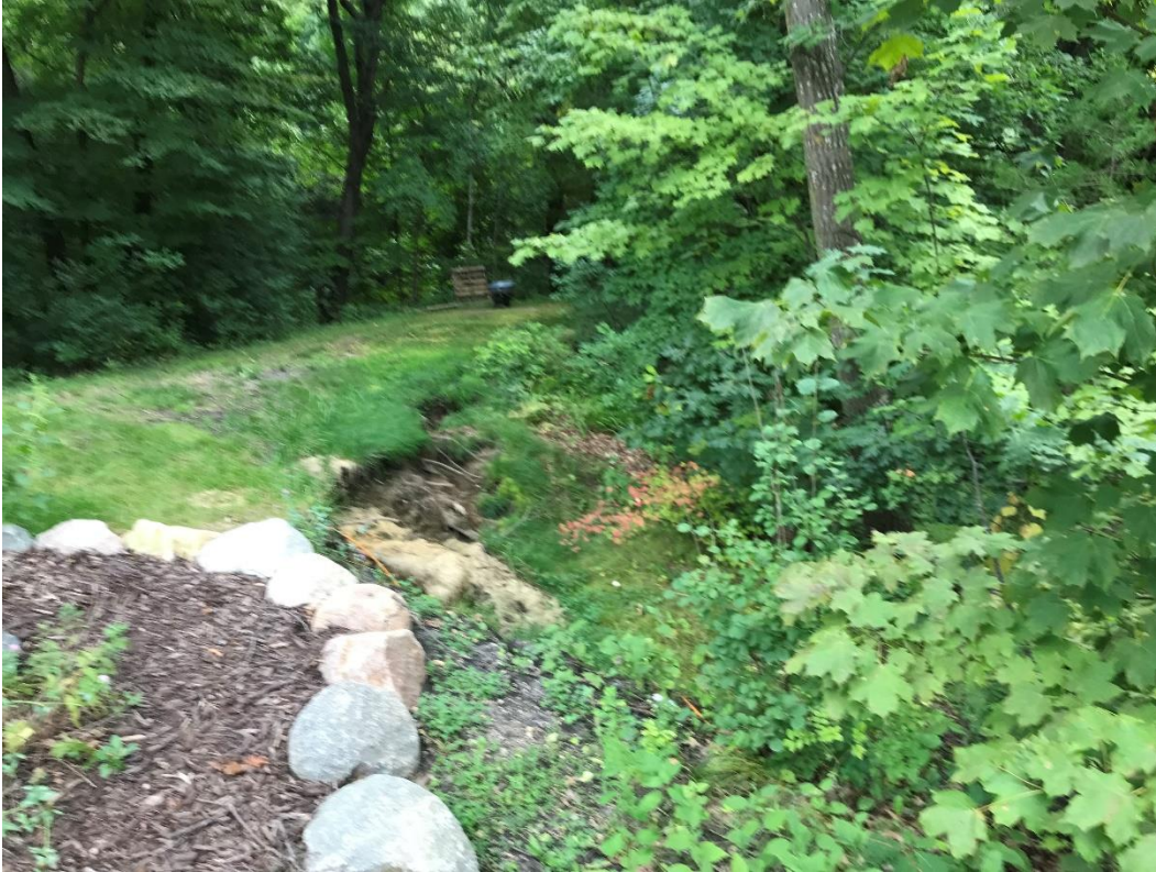
Figure 4. Observed Slope Failure Looking to South End of Failure
