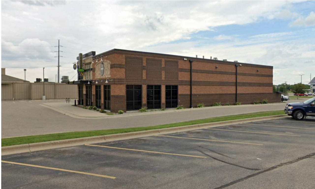
SE VIEW - EXISTING BUILDING
