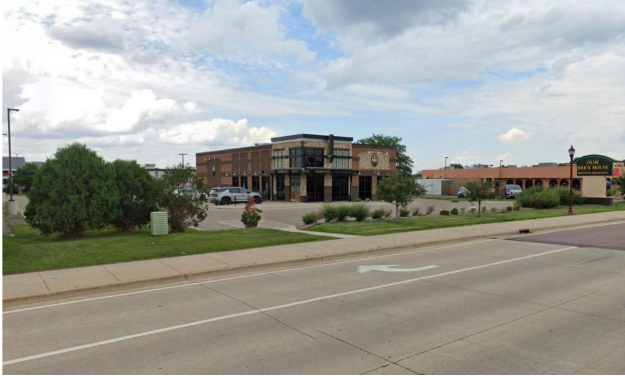
SW VIEW - EXISTING BUILDING
