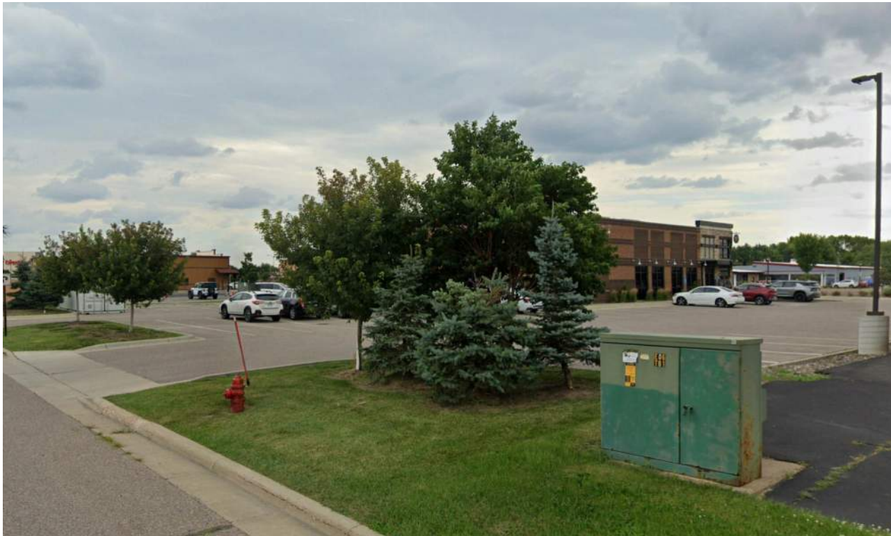
NW VIEW - EXISTING BUILDING
