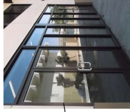
ALUMINUM STOREFRONT FRAMING SYSTEM TUBELITE T14000 DARK BRONZE
