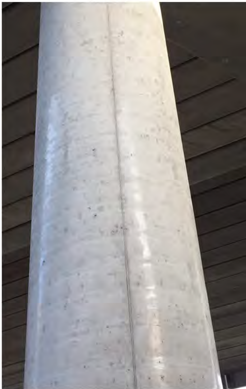
EXPOSED CONCRETE ‘F’ Sonotube cast
