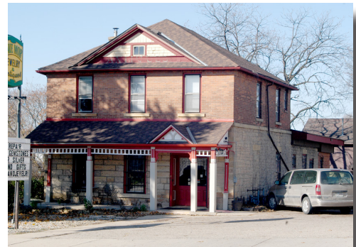
Stone structure at 816 North 2nd Street
