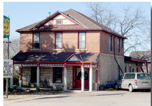
Stone structure at 816 North 2nd Street
