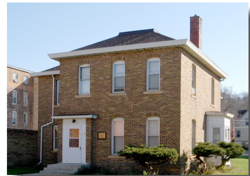
315 South Broad Street
