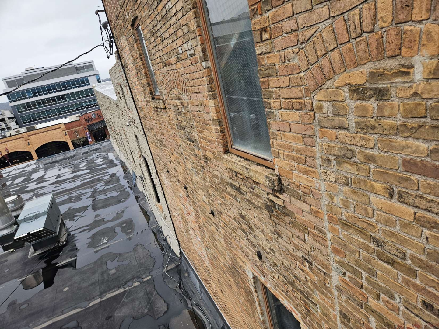
501 S Front Street – Remove Paint, Tuckpointing & Seal Masonry
