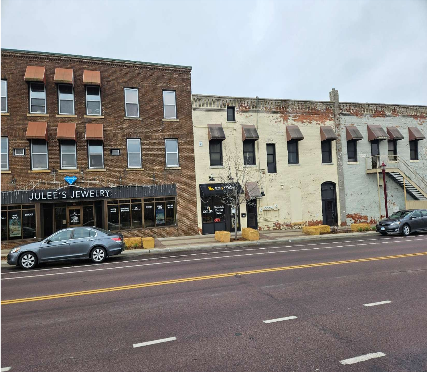
109 E Cherry Street – Tuckpoint & Seal Masonry.
