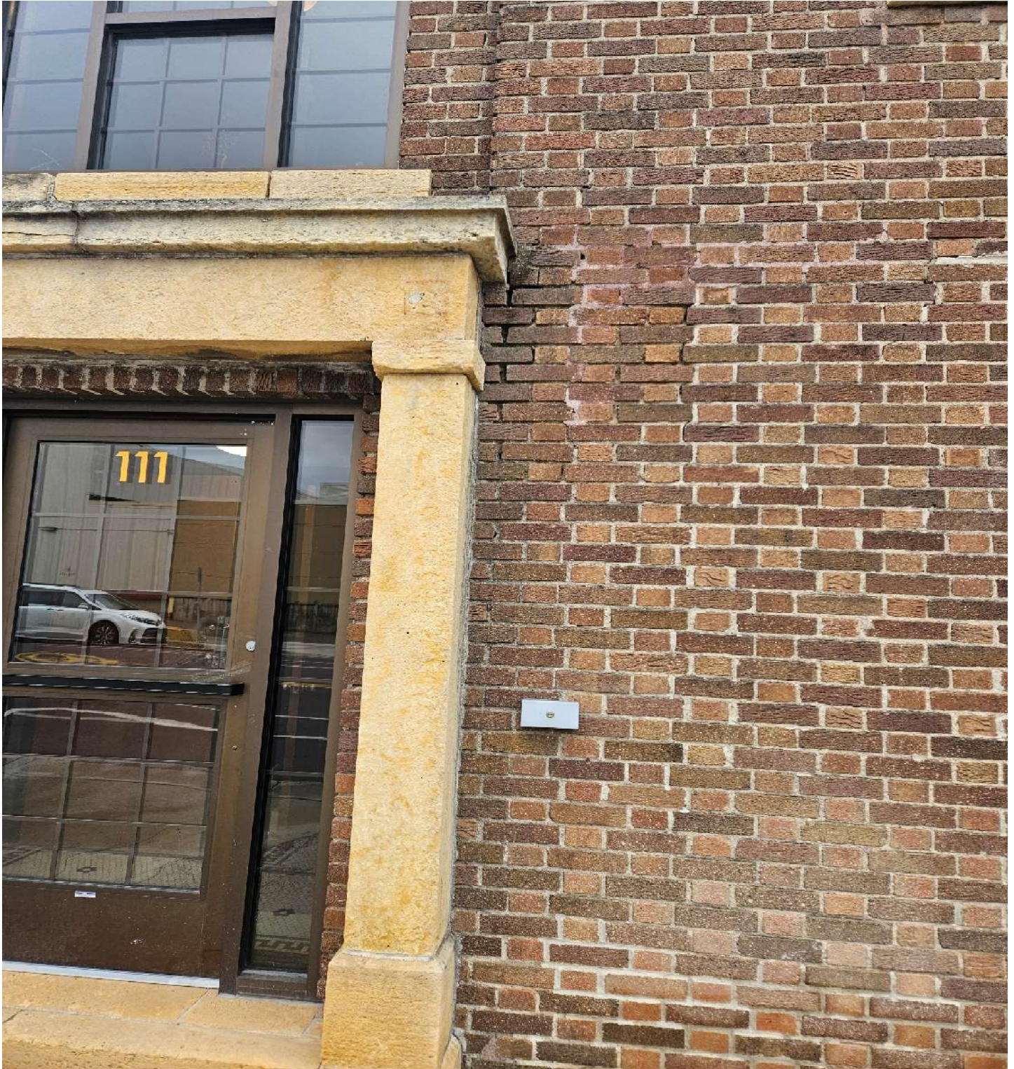
109 E Cherry Street – Tuckpoint & Seal Masonry.
