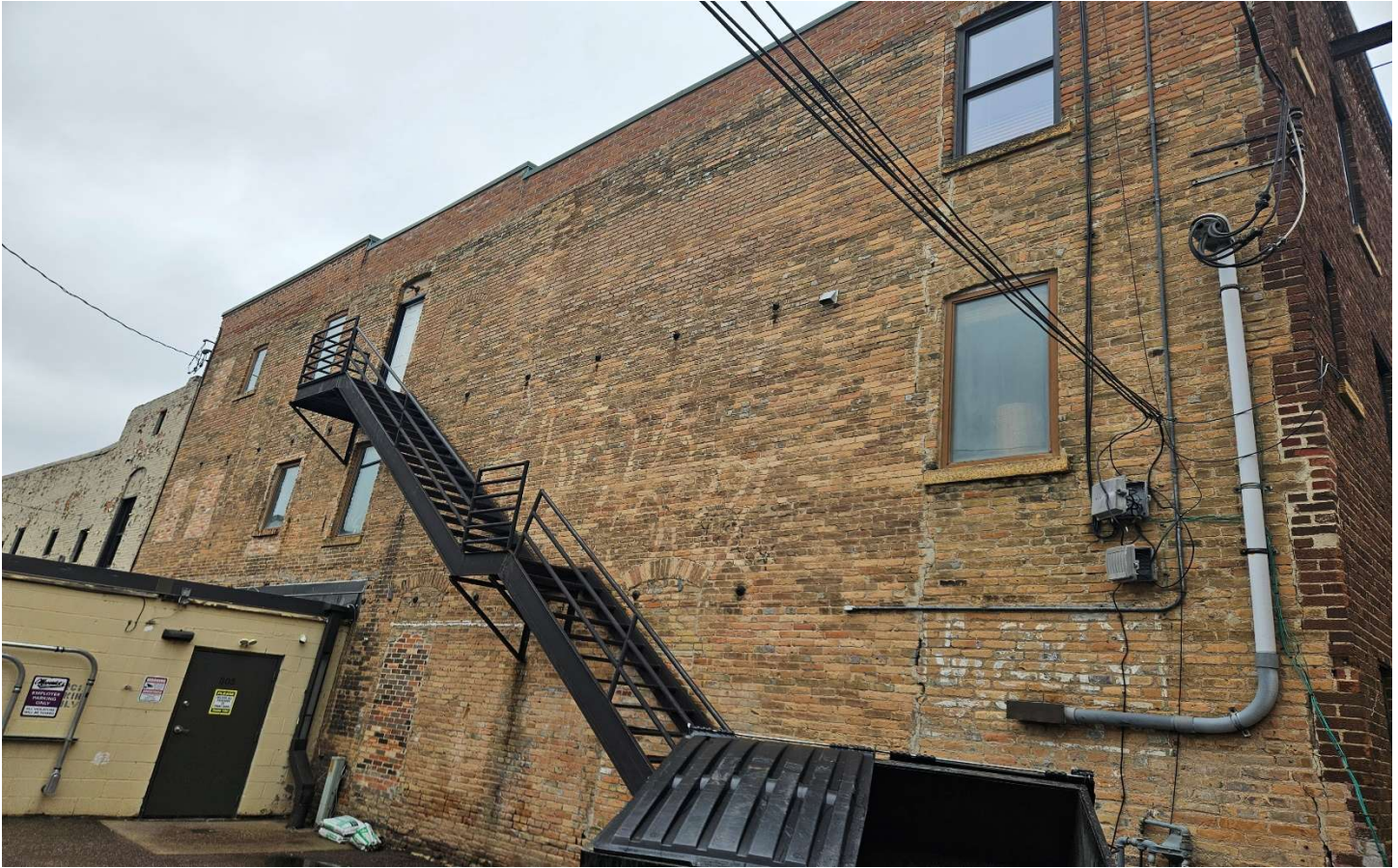
109 E Cherry Street – Tuckpoint & Seal Masonry.
