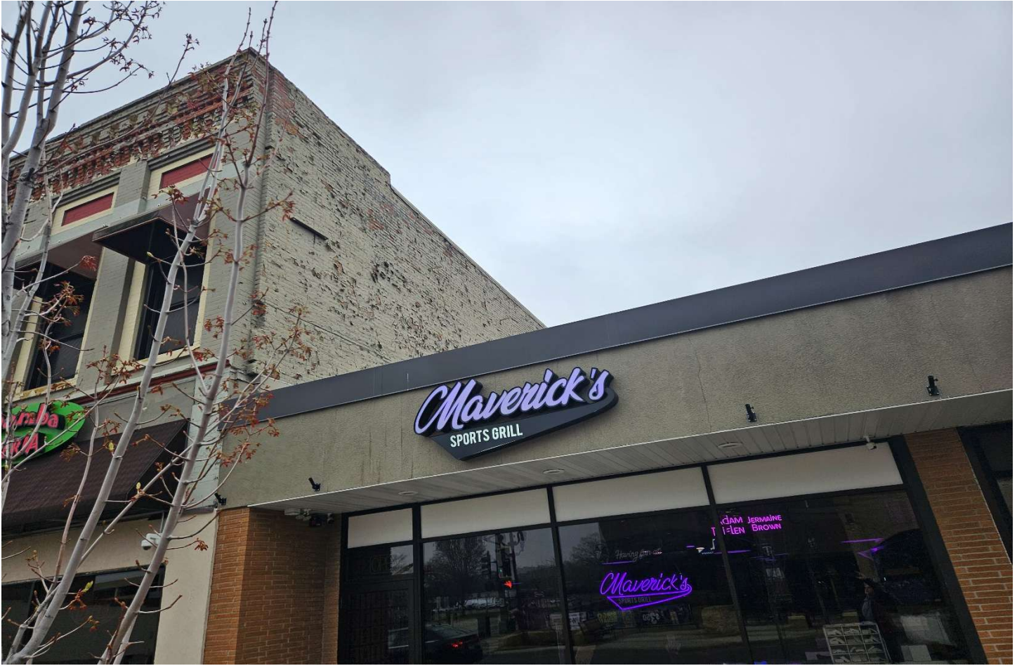
501 S Front Street – Remove Paint, Tuckpointing & Seal Masonry
