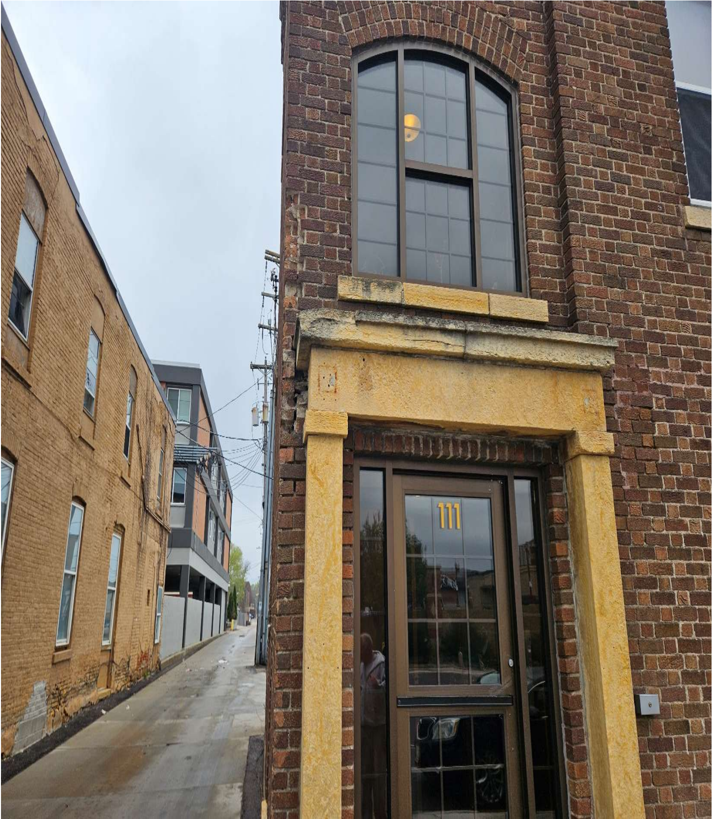
109 E Cherry Street – Tuckpoint & Seal Masonry.
