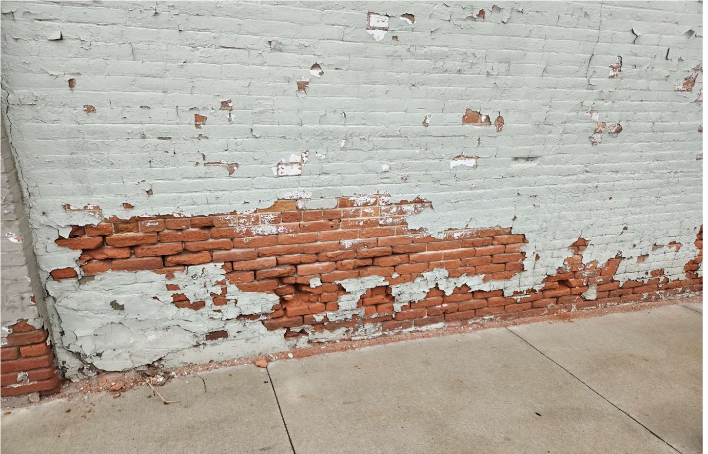
501 S Front Street – Remove Paint, Tuckpointing & Seal Masonry
