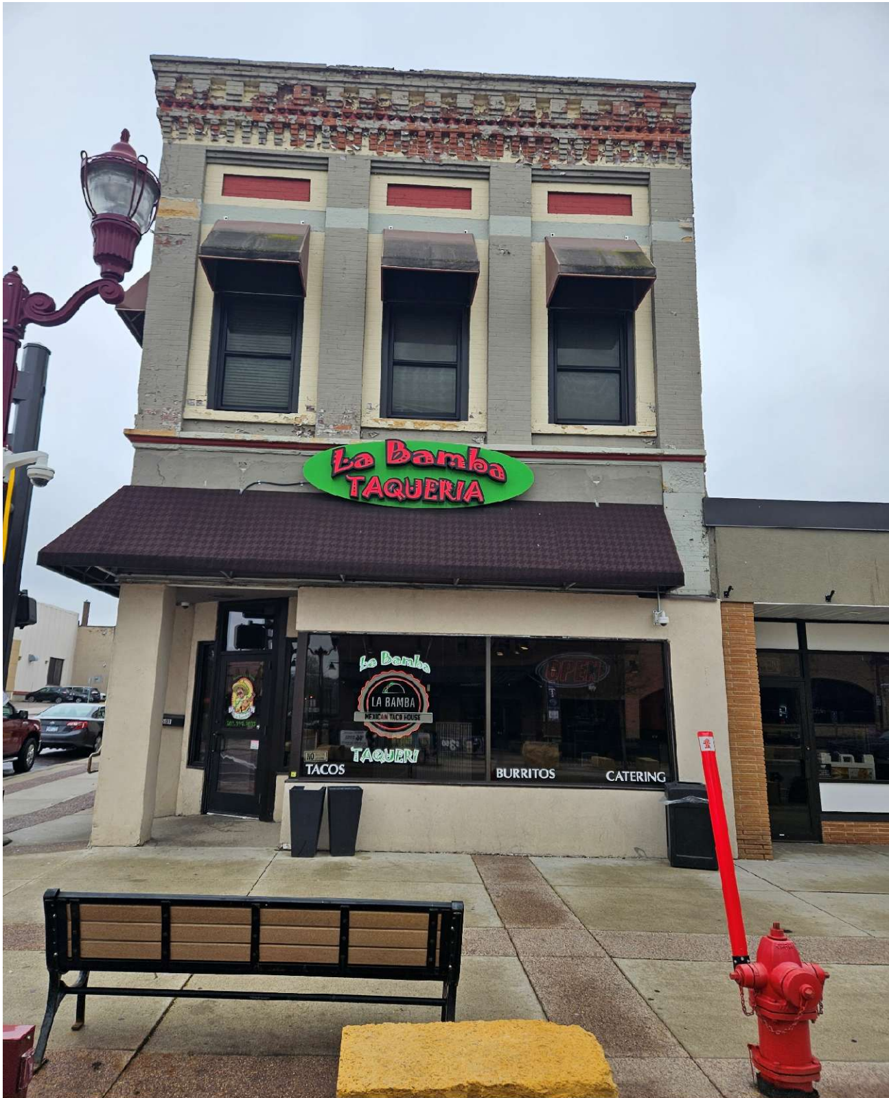
501 S Front Street – Remove Paint, Tuckpointing & Seal Masonry
