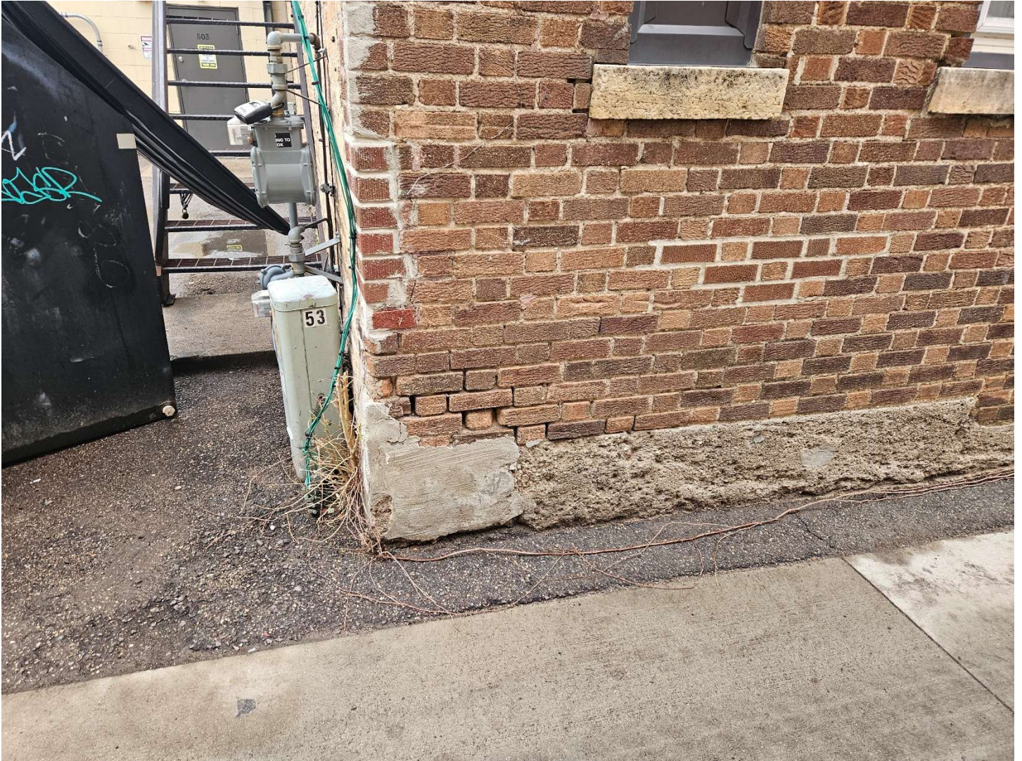
109 E Cherry Street – Tuckpoint & Seal Masonry.
