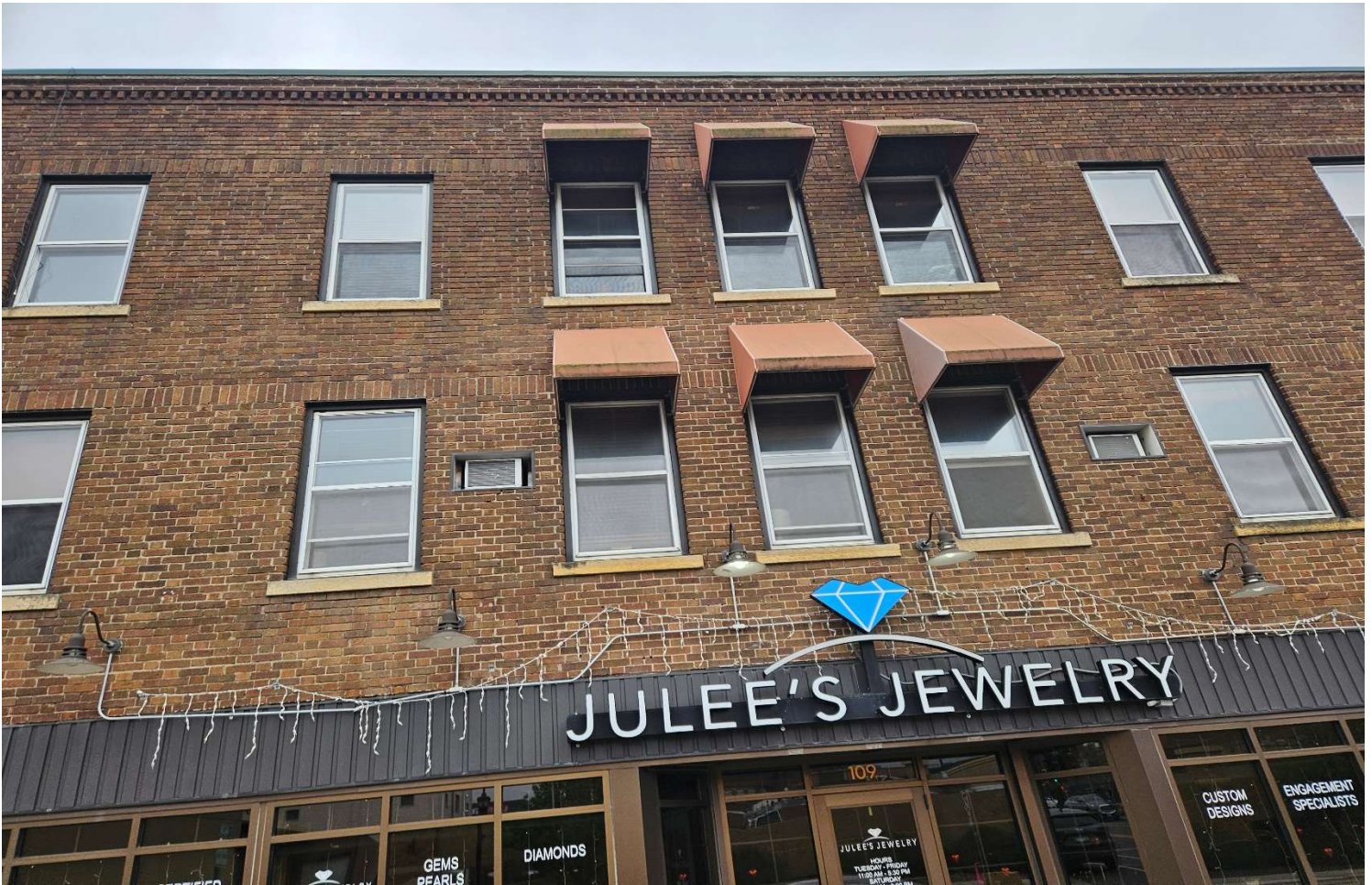
109 E Cherry Street – Tuckpoint & Seal Masonry.
