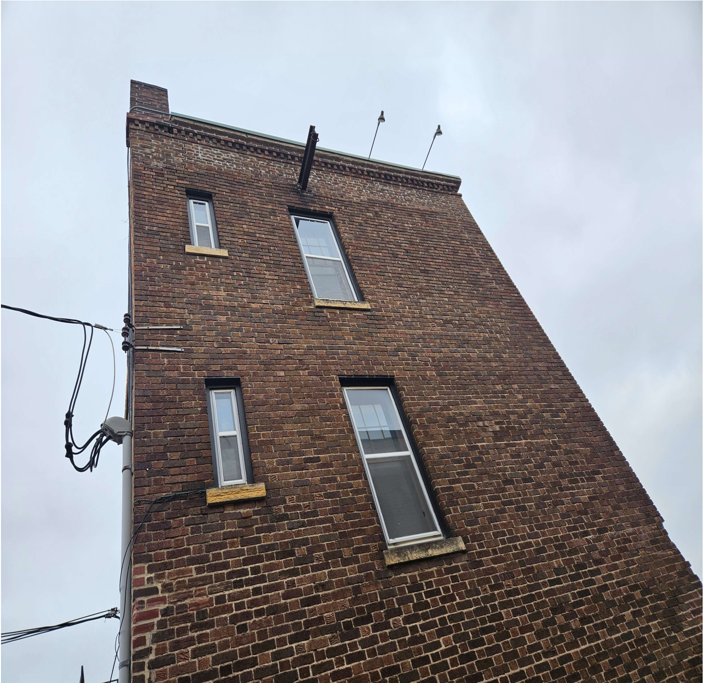
109 E Cherry Street – Tuckpoint & Seal Masonry.
