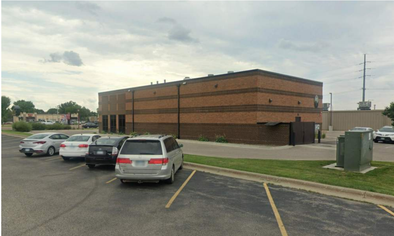
NE VIEW - EXISTING BUILDING
