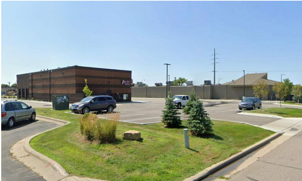
NE VIEW - EXISTING BUILDING
