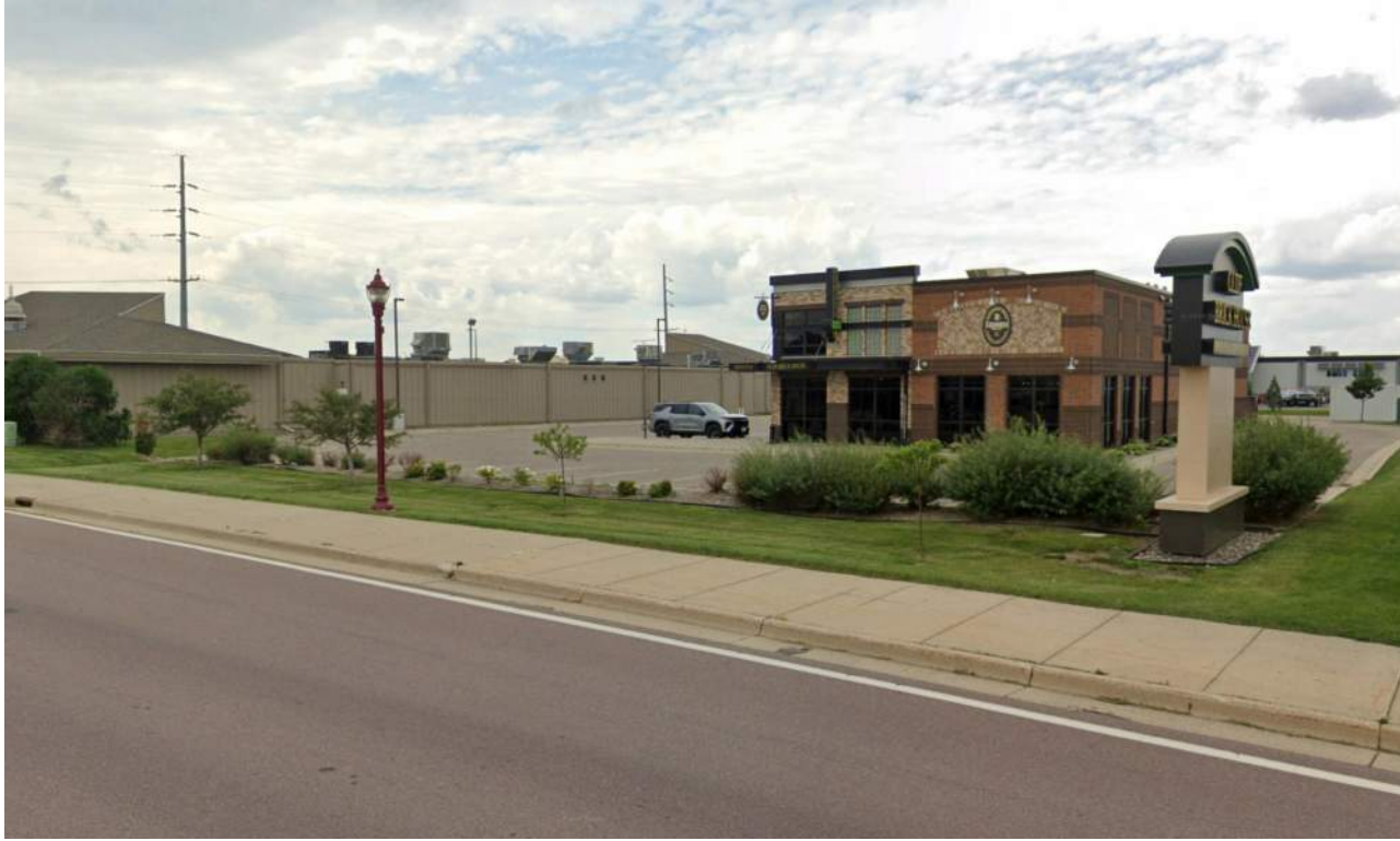
SE VIEW - EXISTING BUILDING
