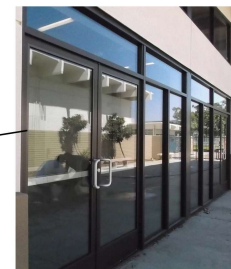
ALUMINUM STOREFRONT FRAMING SYSTEM TUBELITE T14000 DARK BRONZE
