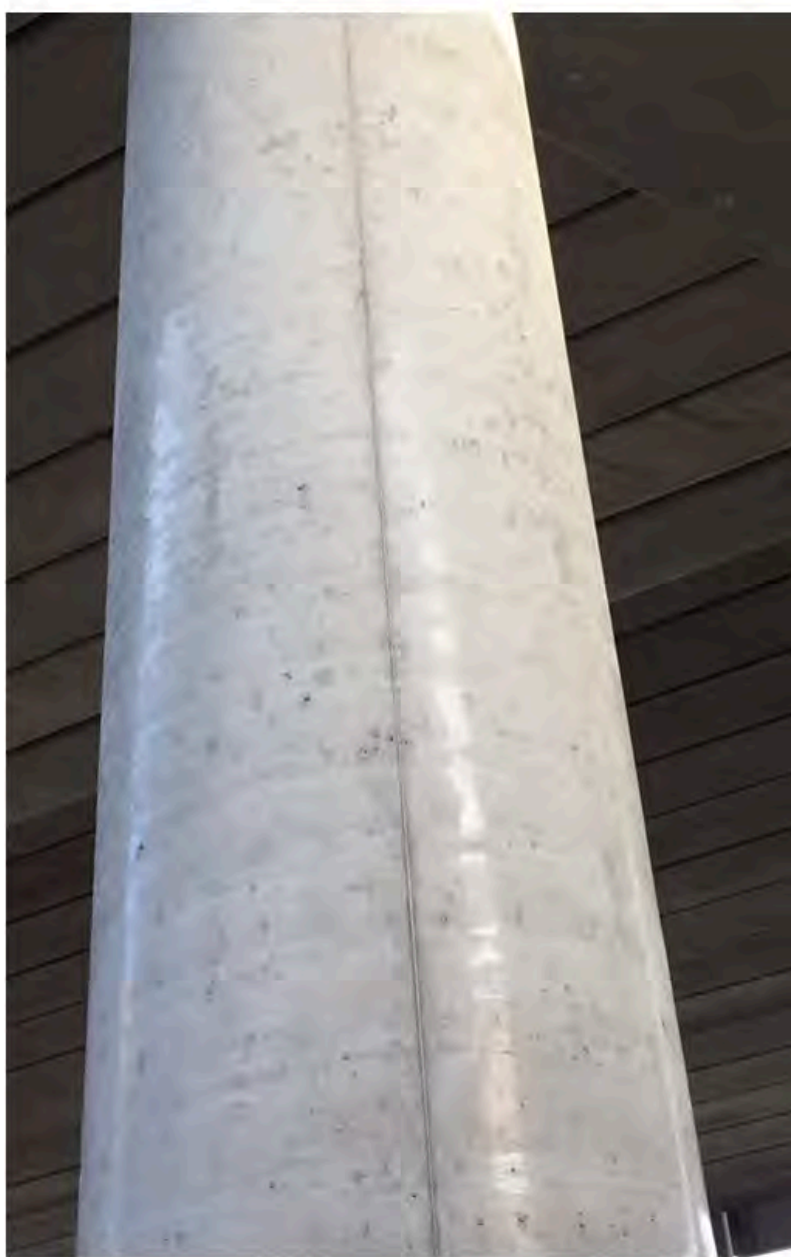
EXPOSED CONCRETE ‘F’ Sonotube cast
