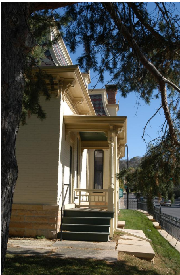
South elevation side porch detail
