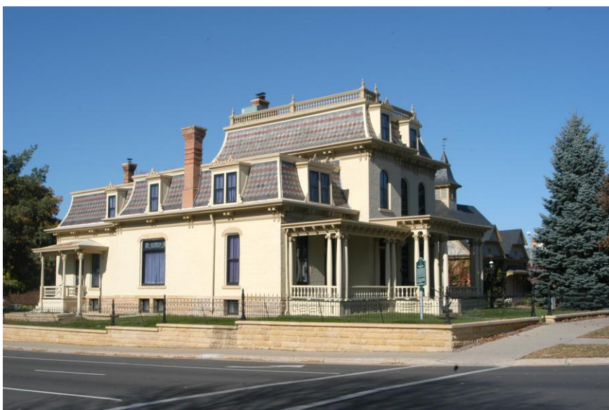
South and east elevations looking northwest
