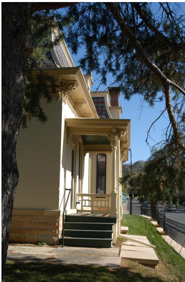
South elevation side porch detail
