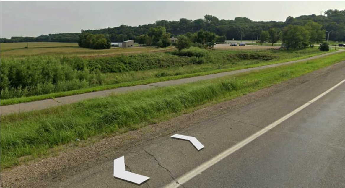
Photo 1 – MnDOT Highway 14 west bound on ramp looking north.
