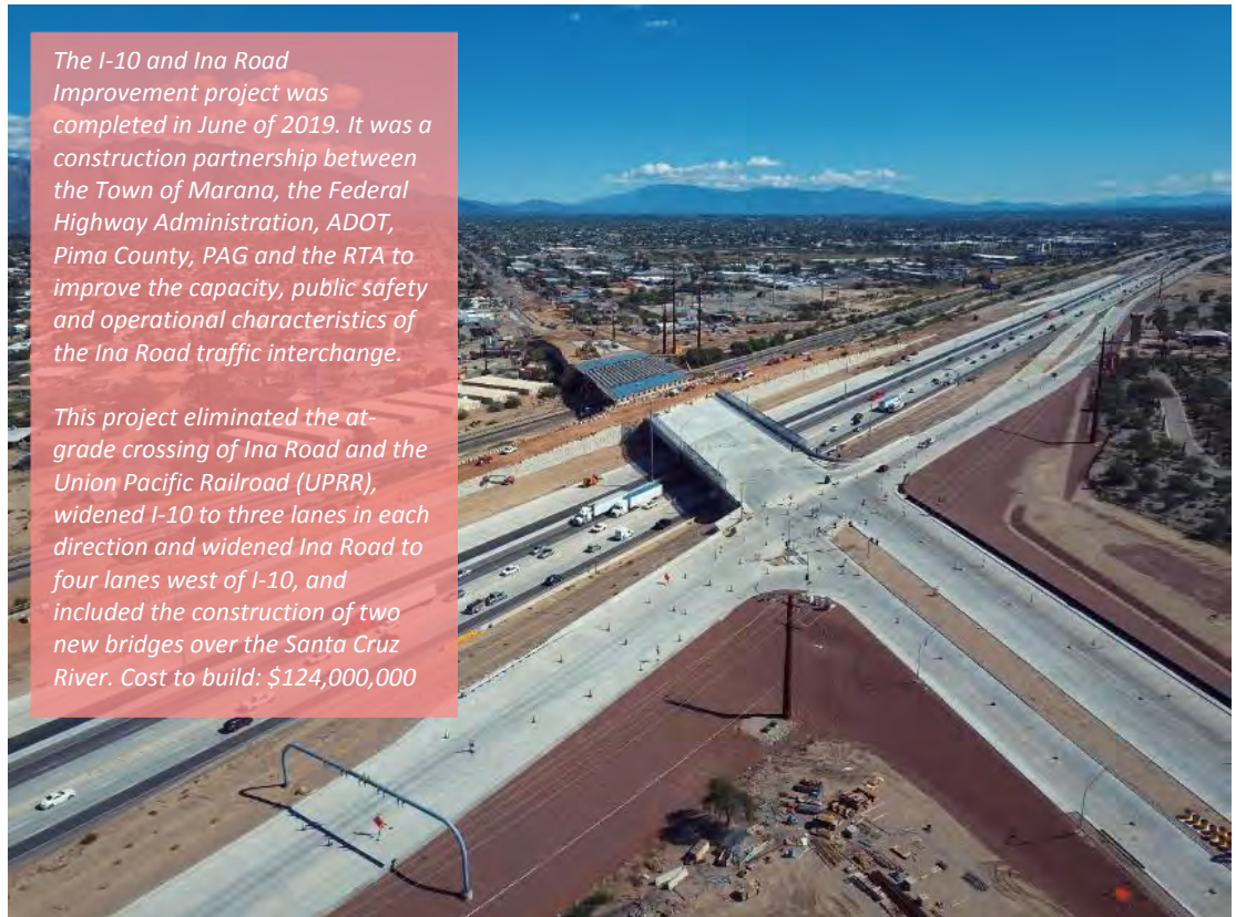
Ina Road construction. Source: Psomas
