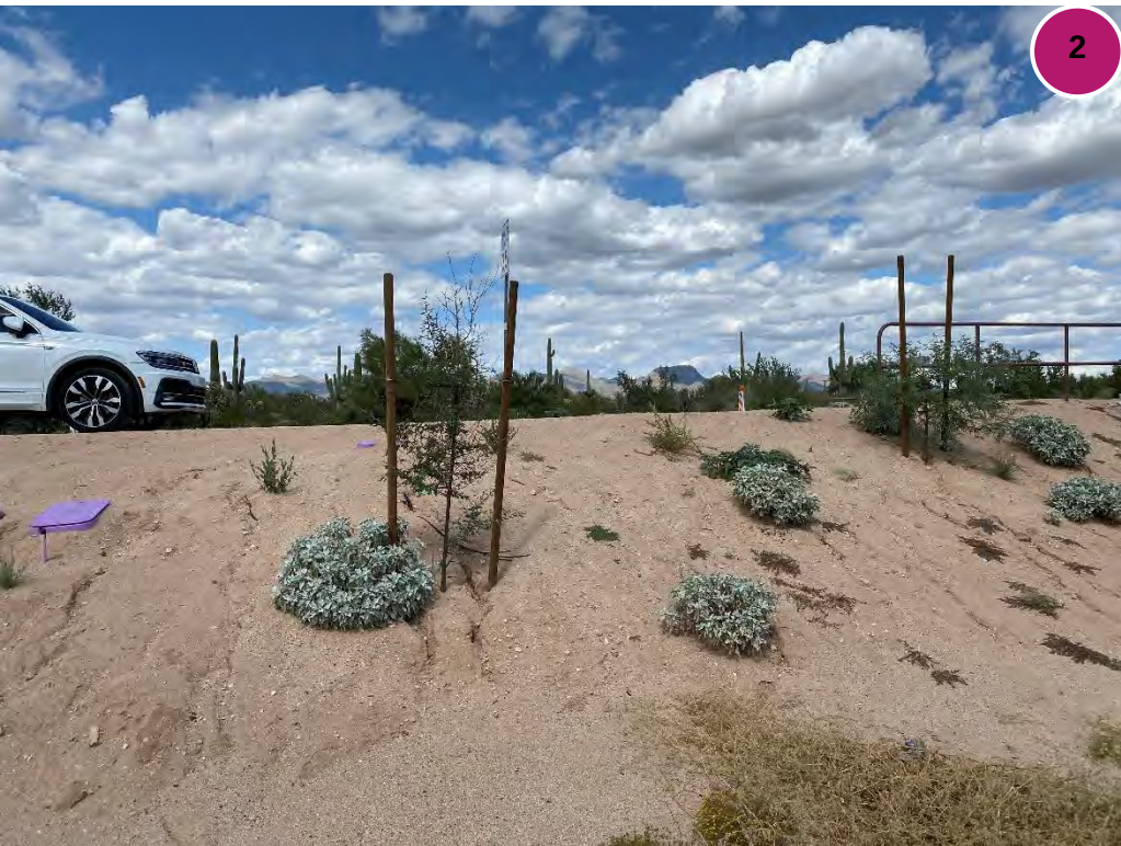
View looking north across Camino de Mañana directly west of the drainage culvert and before the grade change of the roadway obscures northerly views.
