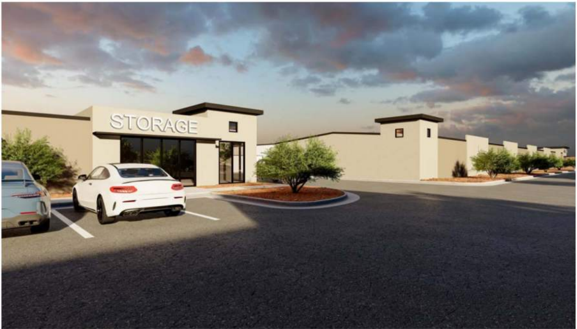
VIEW FACING NORTHEAST FROM INSIDE DEVELOPMENT
