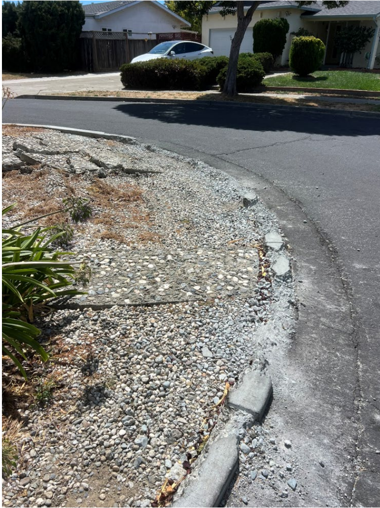
35601 Conestoga Place (cul-de-sac island curb)
