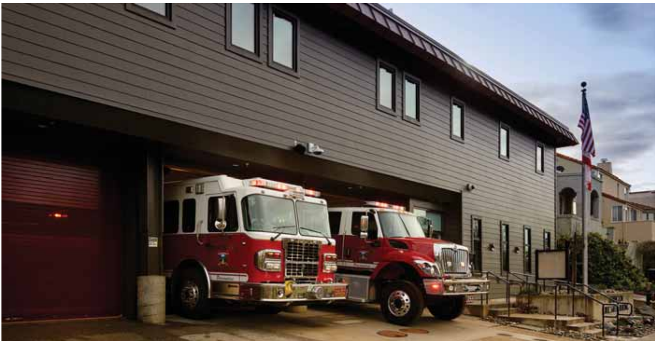
Kensington Fire Protection District Public Safety Building Renovation, Kensington, California | Additional Images
