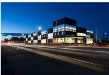
Reach Ashland Youth Center (design-build)
