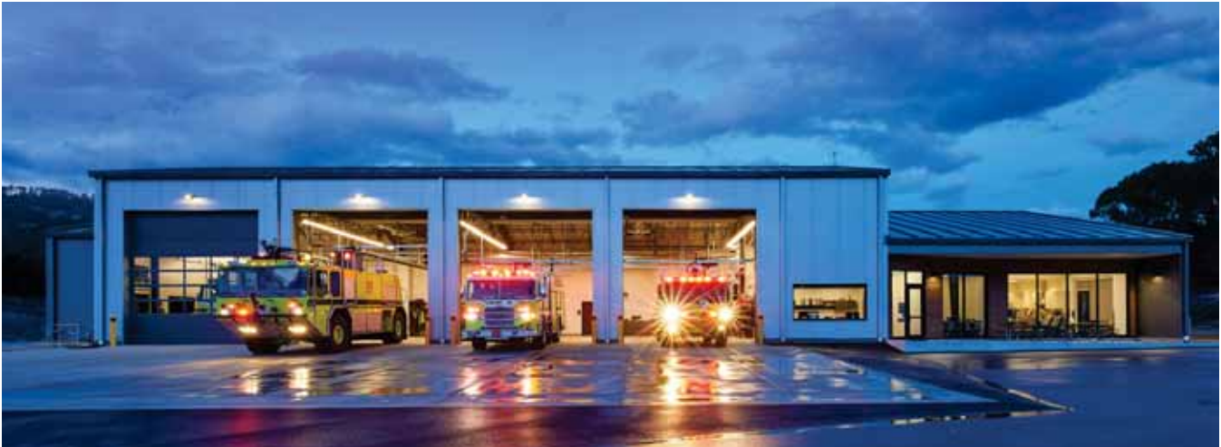
Monterey Regional Airport ARFF Station, Monterey, California | Additional Images
