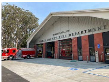
tomales fire station
