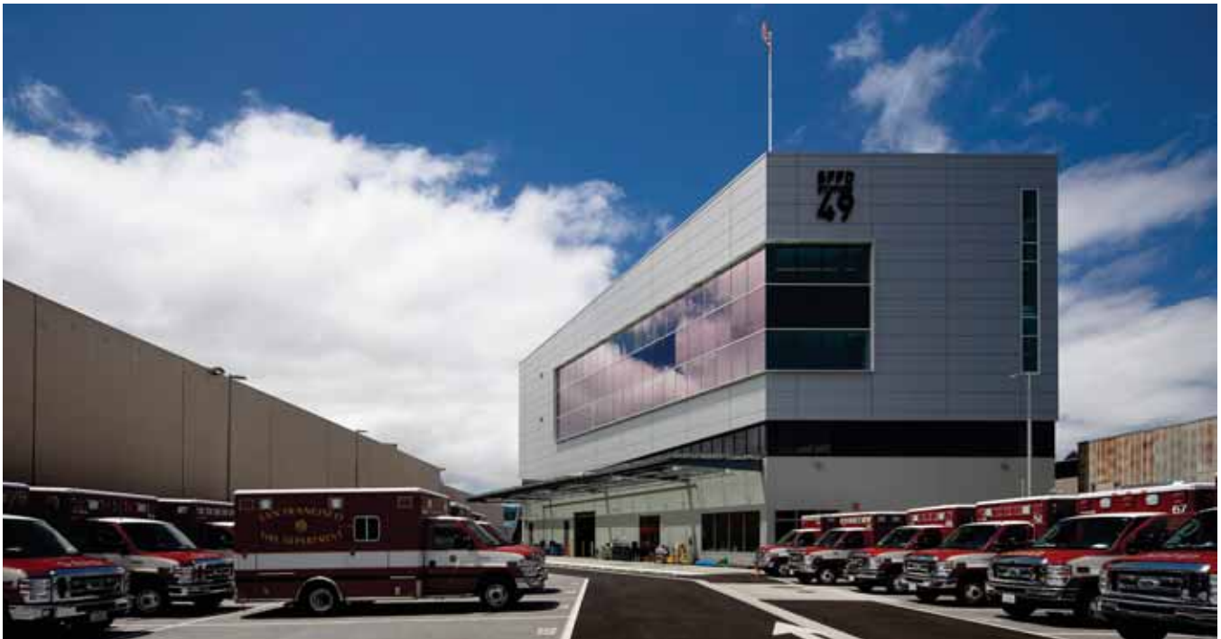
SFFD Ambulance Deployment Facility, San Francisco, California | Additional Images
