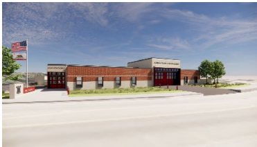
acfd fire station #7 (design-build)
