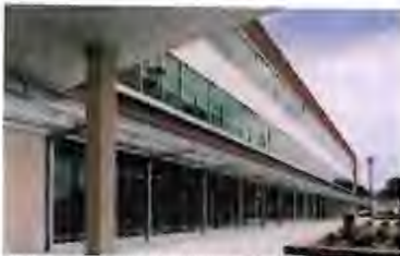
richmond city hall & eoc (design-build)
