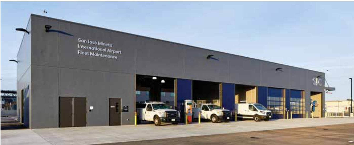
SJC Facilities Administration, Shops, & Fleet Maintenance Buildings, San Jose, California | Additional Images
