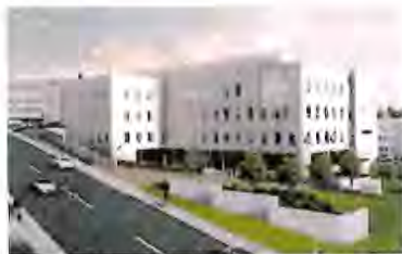
highland hospital acute tower replacement (design-build)
