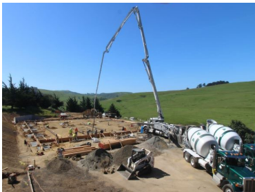
tomales fire station (construction phase)
