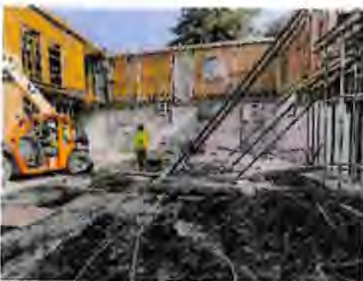
Kensington fire station (construction phase)
