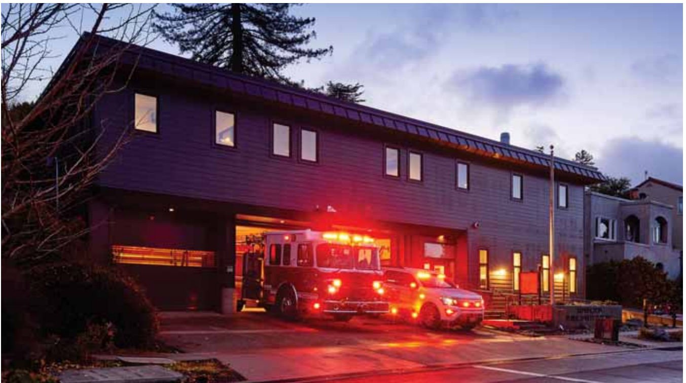
Kensington Fire Protection District Public Safety Building, Kensington, California
