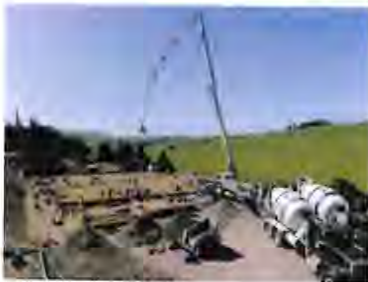
Tomales fire station (construction phase)
