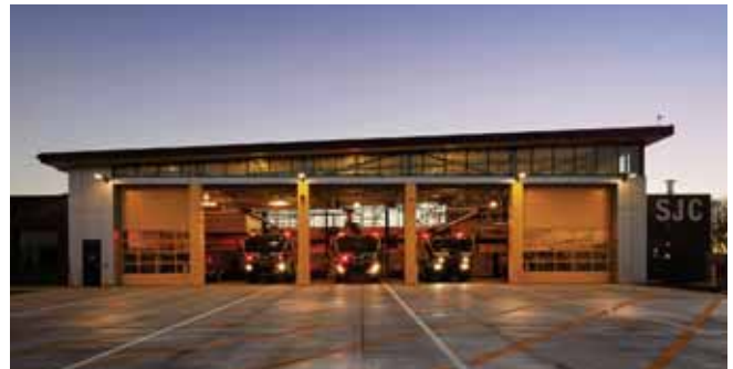
SJC Aircraft Rescue & Fire Fighting (ARFF) Station 20, 2022
