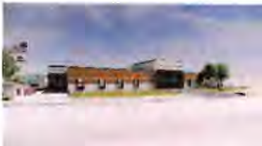
acfd fire station #7 (design-build)
