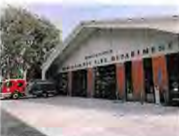
tomales fire station
