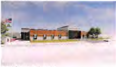
acfd fire station #7 (design-build)
