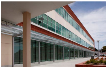
richmond city hall & eoc (design-build)
