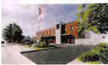
acfd fire station #25 (design-build)
