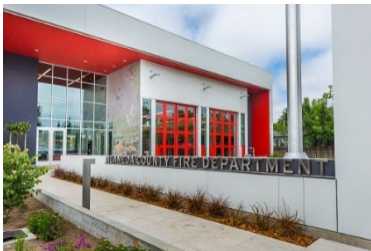
acfd cherryland fire station #23
