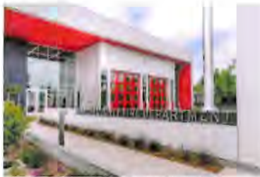
acfd cherryland fire station #29
