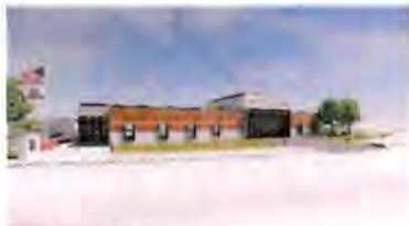
acfd fire station #7 (design-build)
