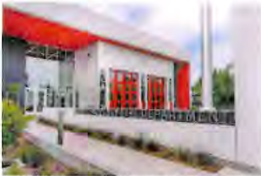
acfd cherryland fire station #23
