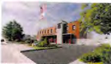
acfd fire station #25 (design-build)
