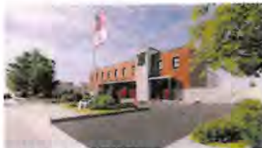
acfd fire station #25 (design-build)
