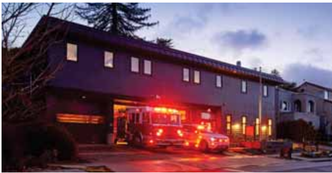
Kensington Public Safety Building Renovation, 2025
