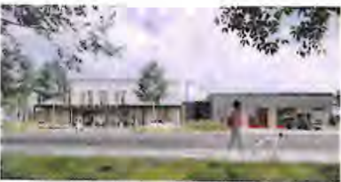
petaluma public safety facility with fire station & eoc (design-build)
